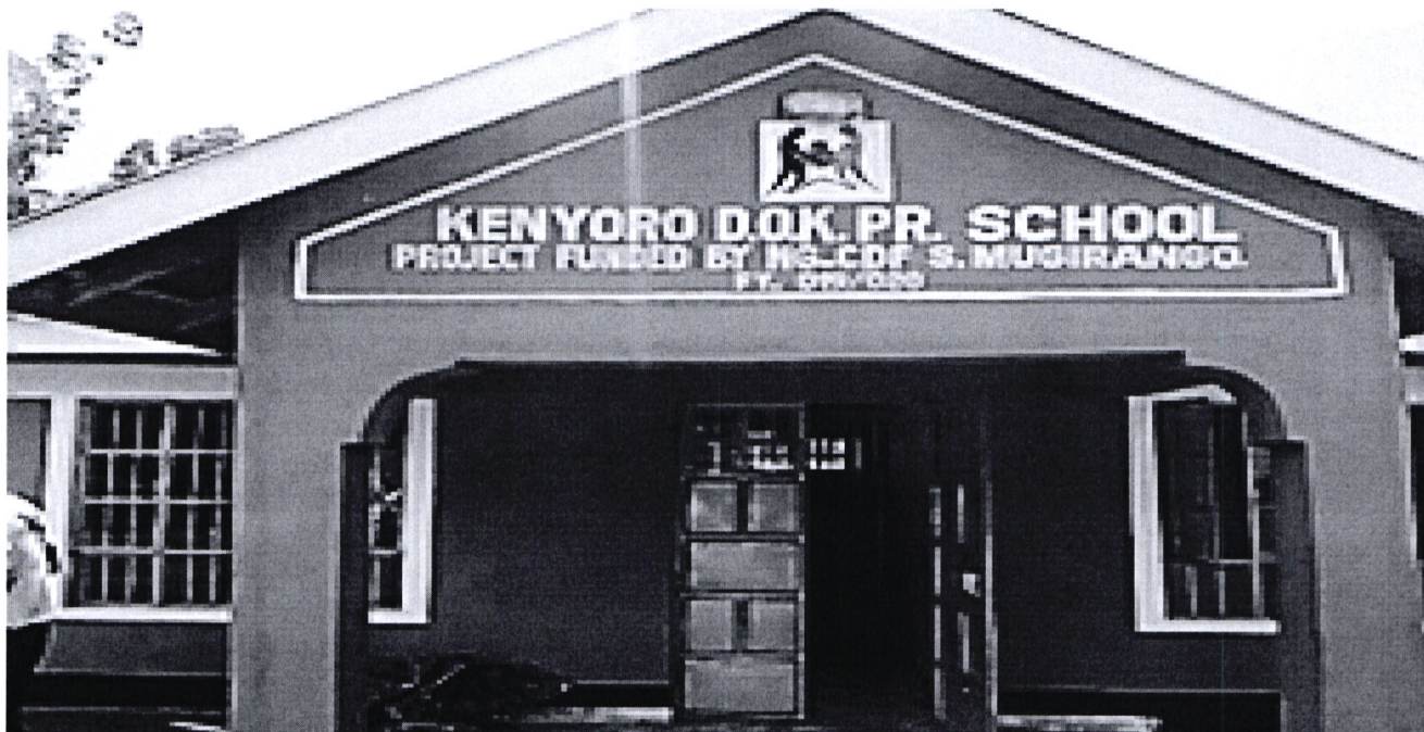
Kenyoro primary School –Completion of Administartion Office.
