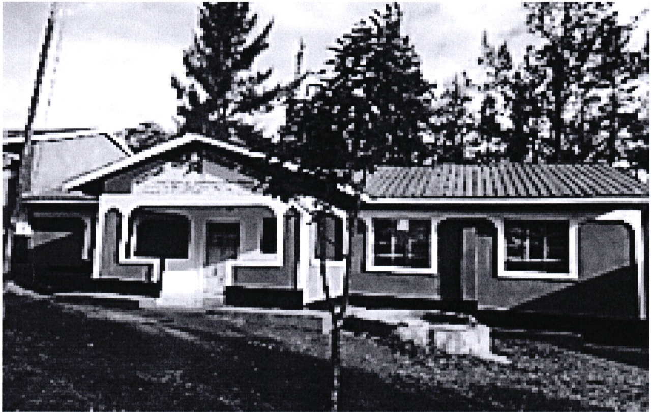
Gesonso Primary School – Completion of administration office
