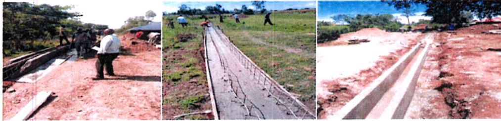
Damlo General Contractors working on block BR 4 Kimira Scheme Lot 6
