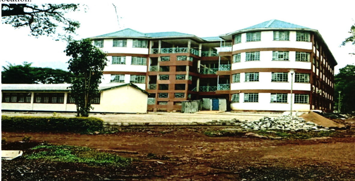
Figure 4: The Education Complex that is at 98% completion and should be in use by early 2019 to address the critical shortage of training facilities at the College
