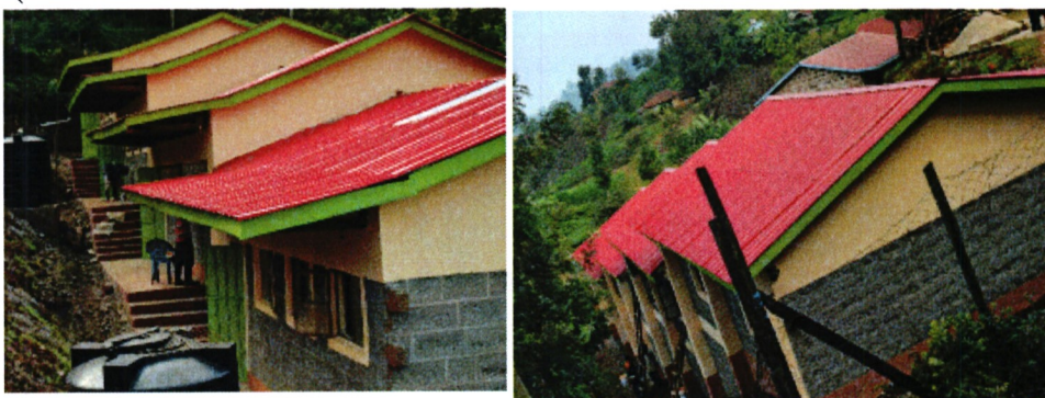
Nge-ini Primary School-Renovation of Classrooms 2020/2021
