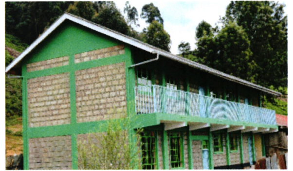
Gachogi Pry Sch-Construction of four classrooms 2 Storeyed
