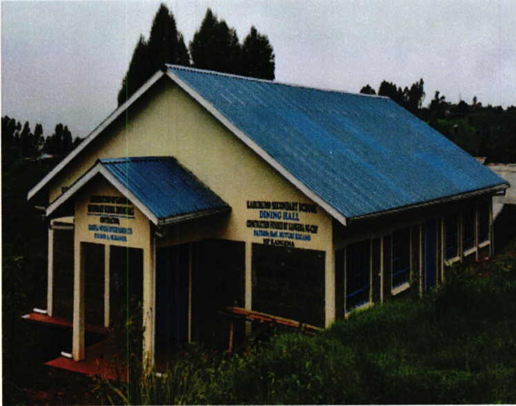
Karurumo Sec School-Dining Hall Construction
