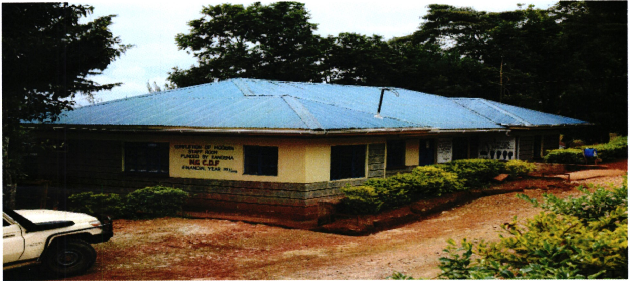
Githiga Primary School-Construction of a Model Staffroom
