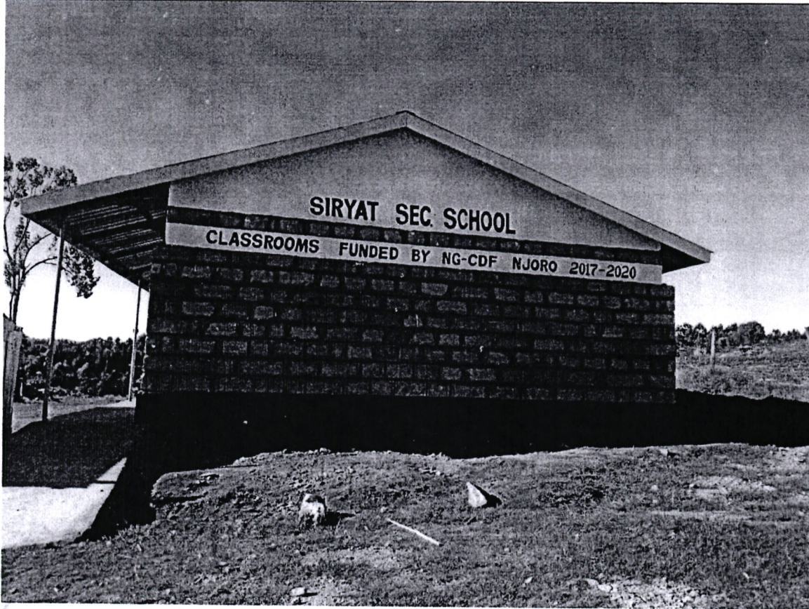
FIG 1.1 CONSTRUCTION OF TWO CLASSROOMS TO COMPLETION
