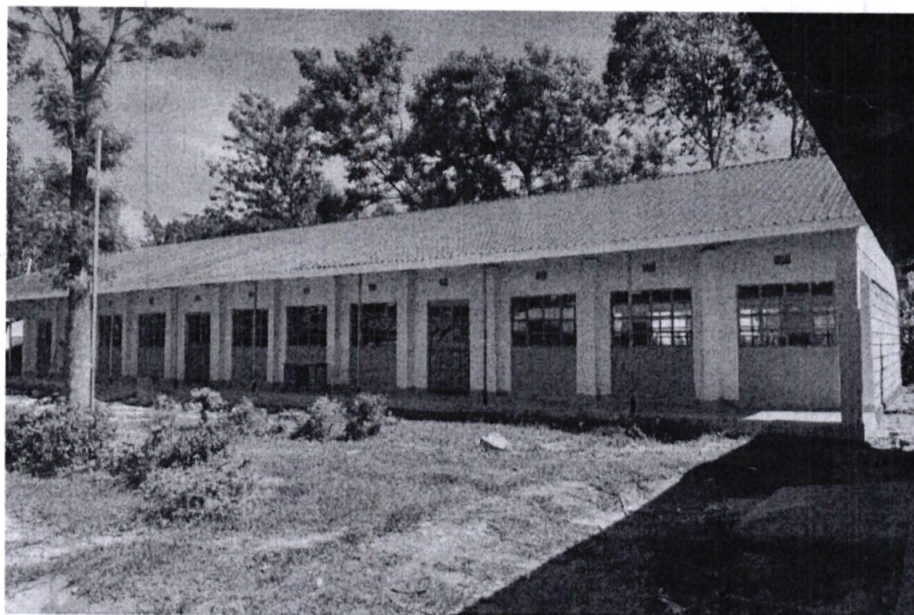
Buhayi Muslim Primary School-Construction of 3no. Classroom.
