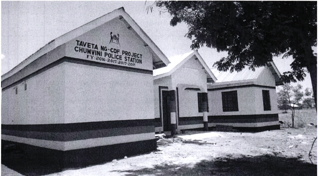
Chumvini Police Station Project
