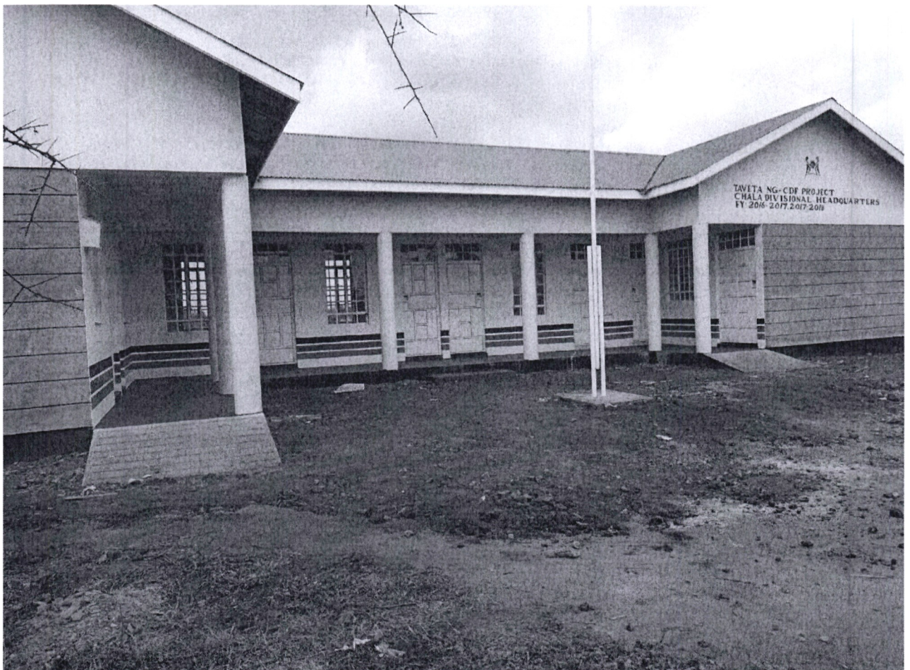
Chala divisional headquarters project
