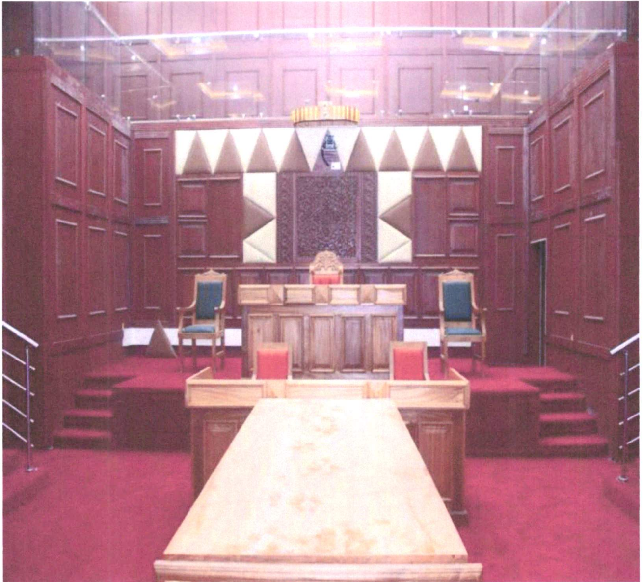
Ongoing construction of ultra-modern chamber for the County Assembly of Marsabit.
