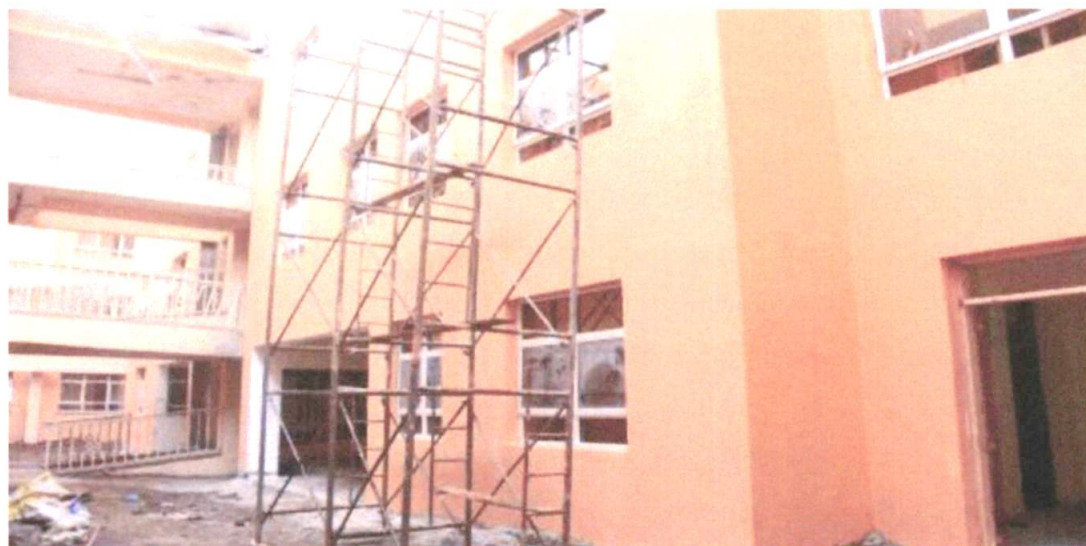
Ongoing construction of extension office block
