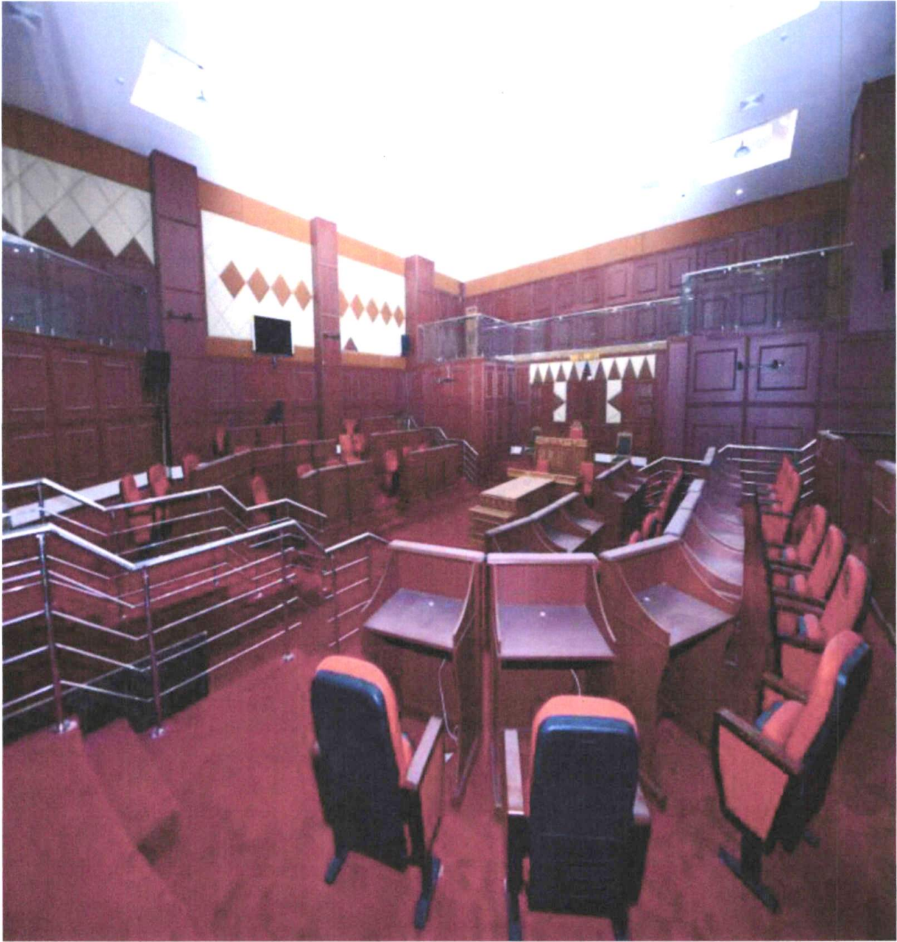
Ongoing construction of ultra-modern chamber for the County Assembly of Marsabit.
