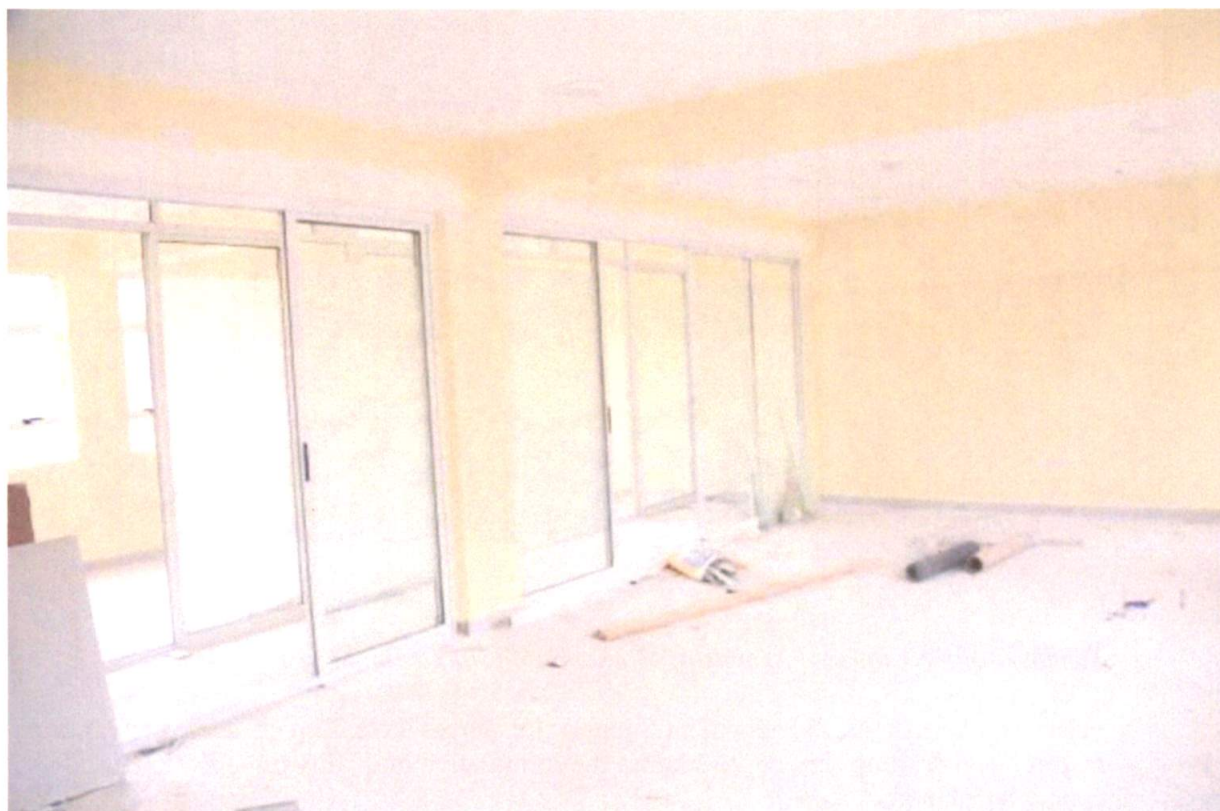
Ongoing construction of modern office block
