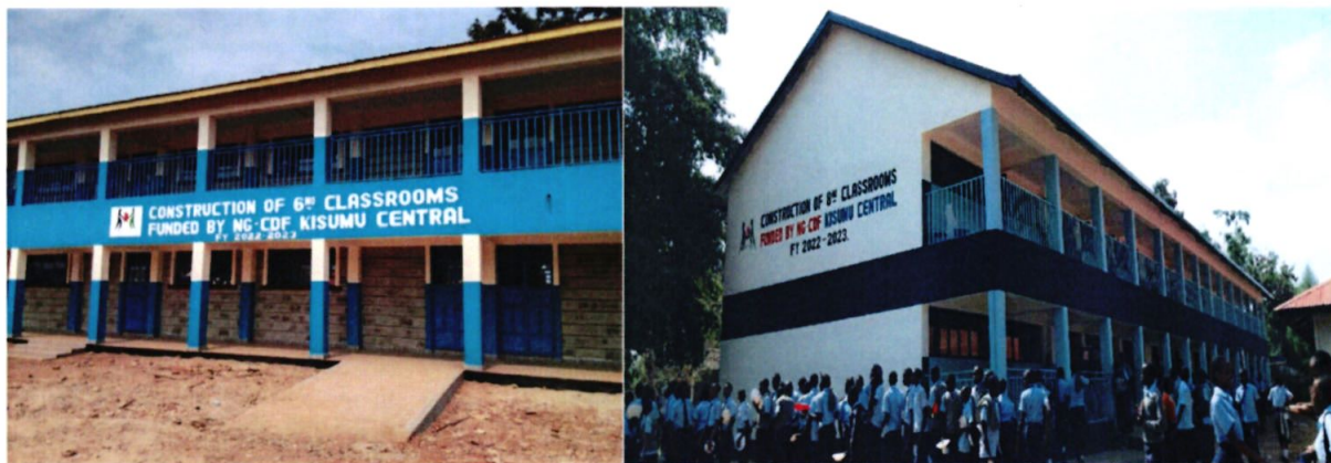
Newly constructed classrooms in Manyatta Primary School and Lions High School
