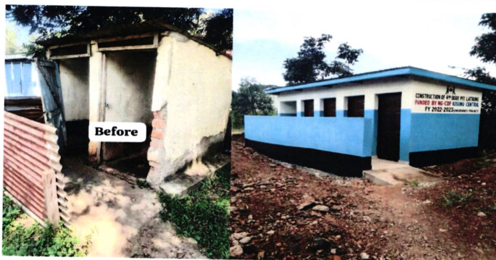
Kisumu Union Primary School 4 door toilet
