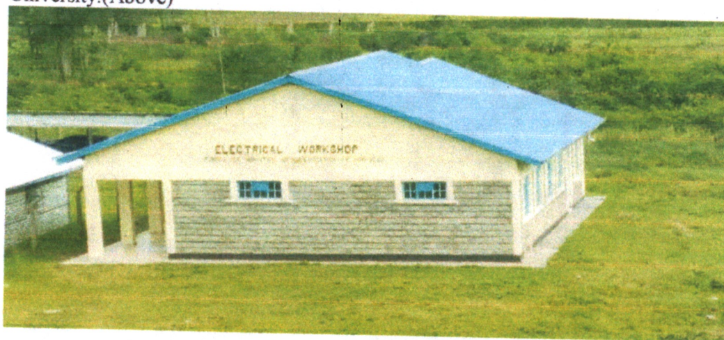
Above. The Electrical Workshop above Funded by GOK through the Ministry of Education now completed.
