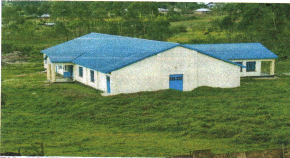
TOP. NG-CDF Rongo Sponsored Dining Hall now complete awaiting handing over
