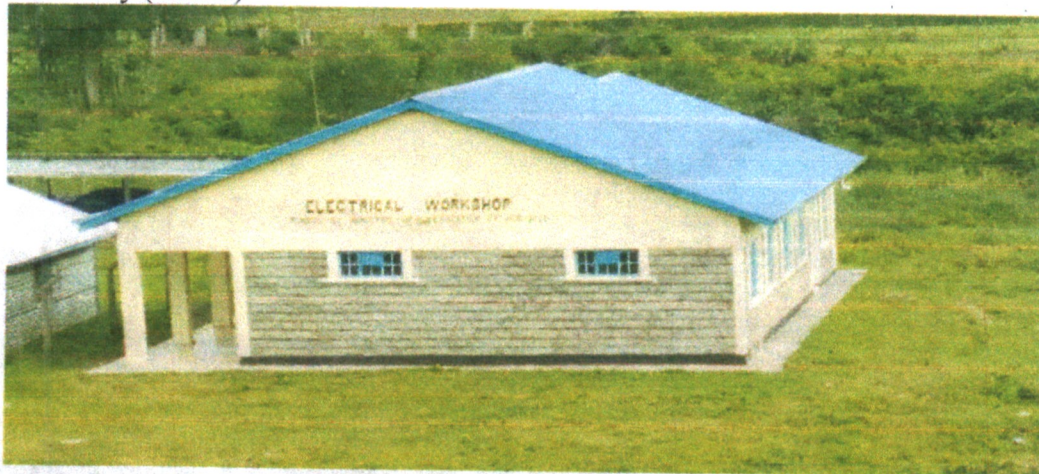
Above. The Electrical Workshop above Funded by GOK through the Ministry of Education now completed.
