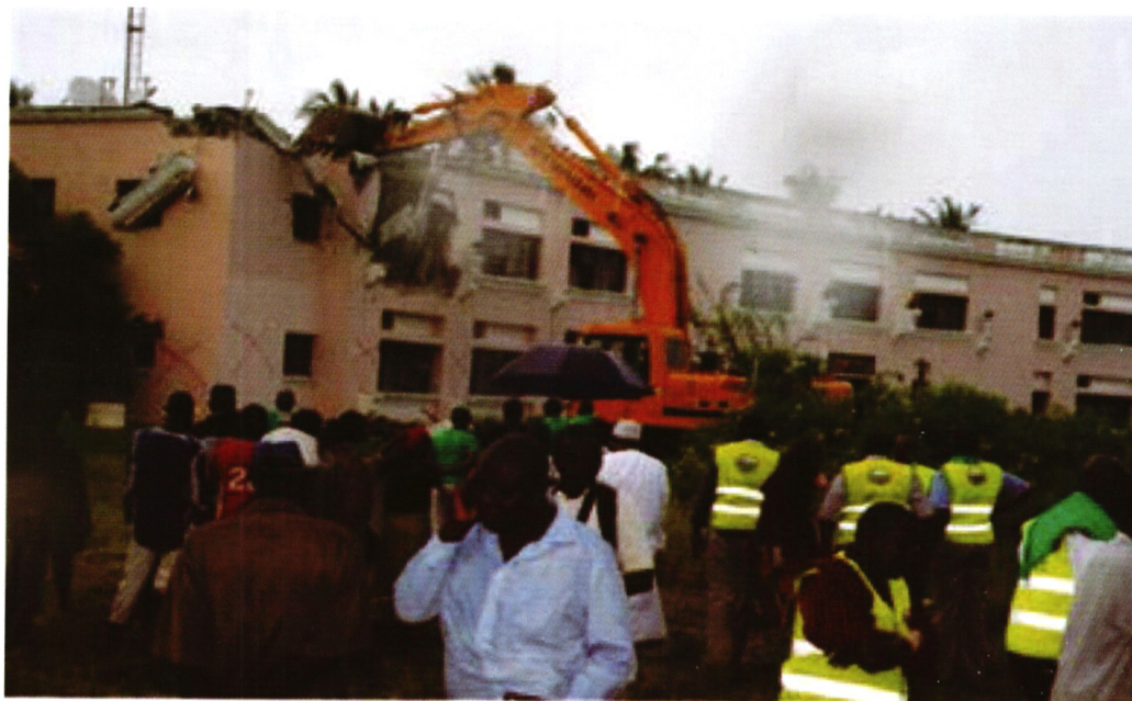
Demolition of the Safari Club Hotel built on a road reserve in Shanzu, Mombasa on 27 th June 2013.
