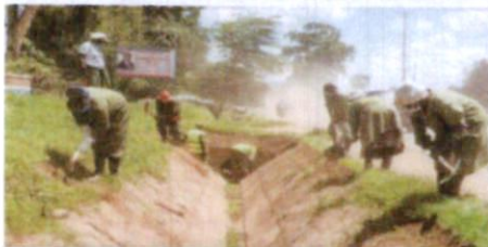
Drainage clean-up, Nanyuki
