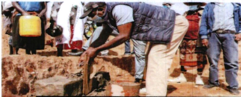
Makuriaan Water Project: Governor lays tank foundation at Arjiu tank
