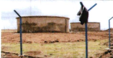
Makurian Water project - Mukogondo East
