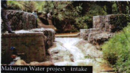
Makurian Water project - intake
