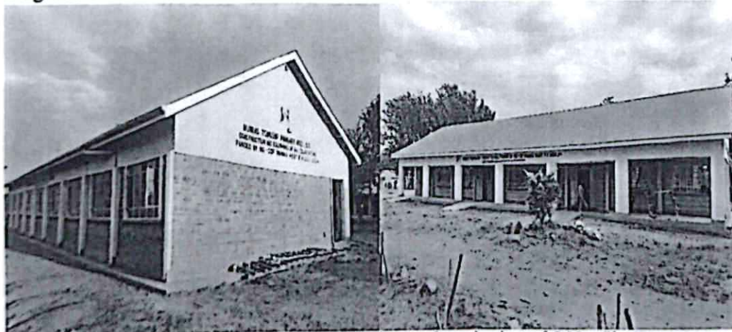
Mumias Township Primary School- Construction and equipping of 3 No. Classrooms
