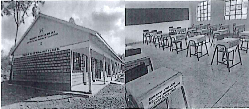
Bumanyi Primary School- Construction and equipping of 3 No. Classrooms
