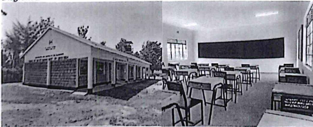
St. Vincent Utende Primary School- Construction and equipping of 3 No. Classrooms
