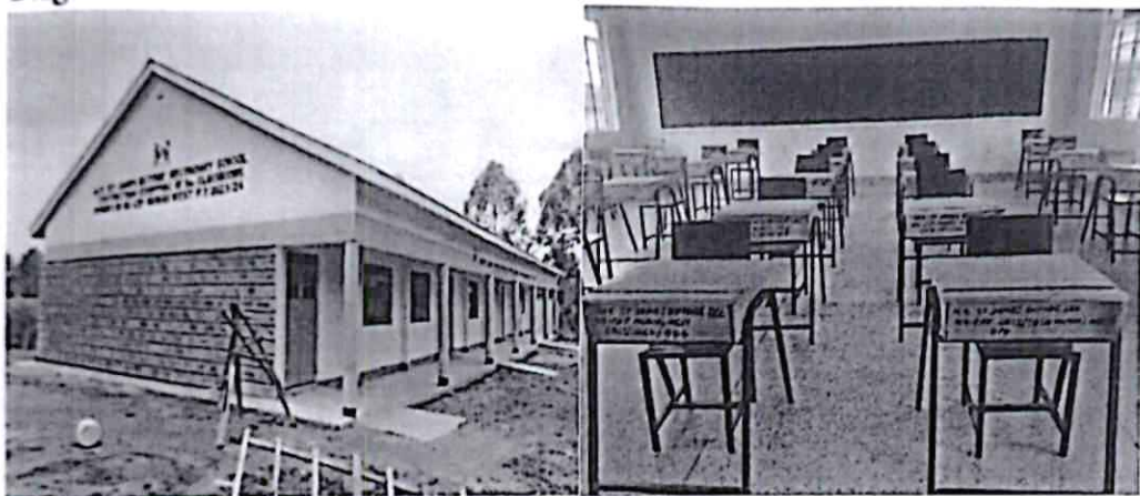
St. James Butobe Secondary School- Construction and equipping of 3 No. Classrooms
