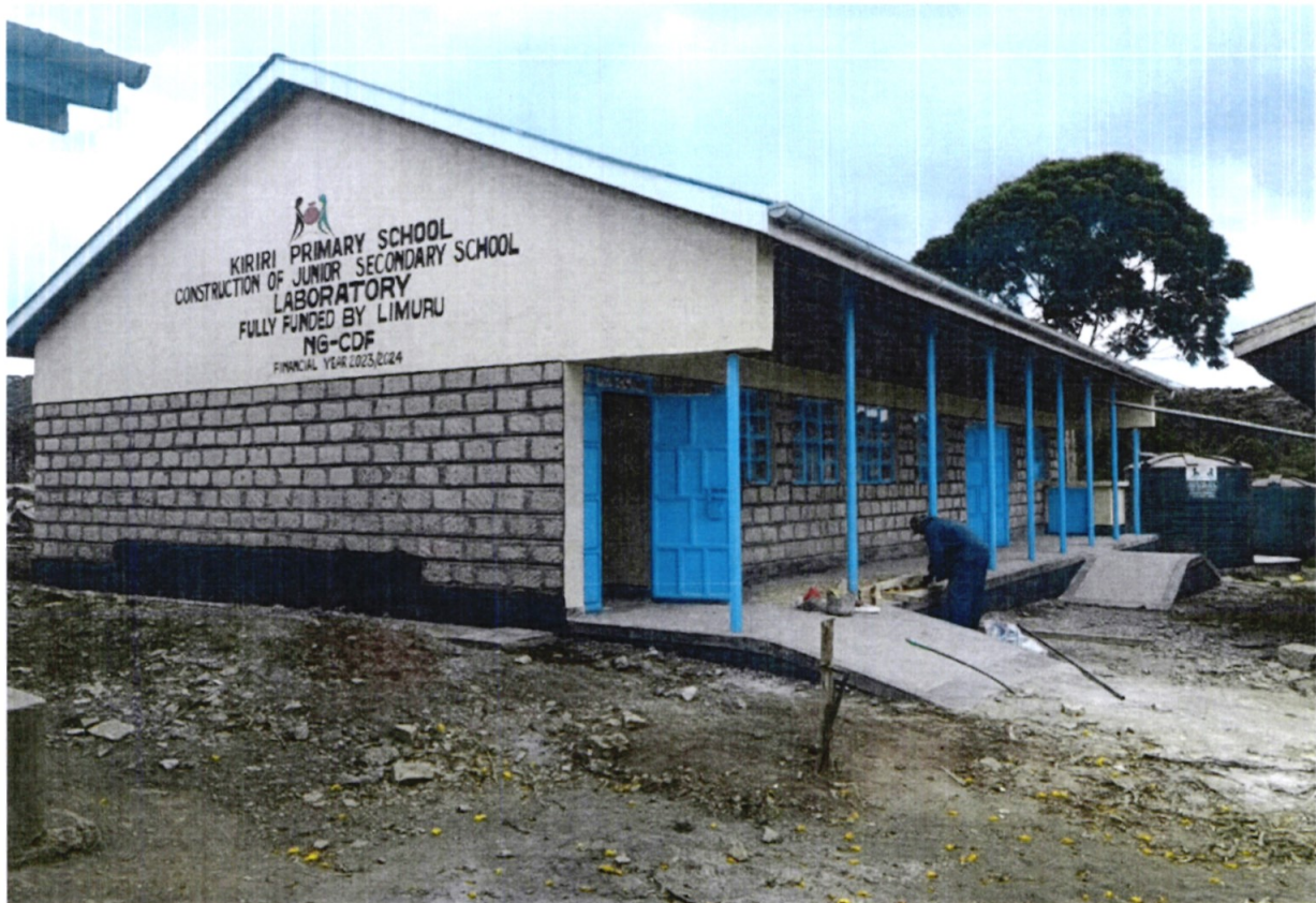
Kiriri Primary and Junior school-Completed 40 capacity Junior Secondary School Laboratory
