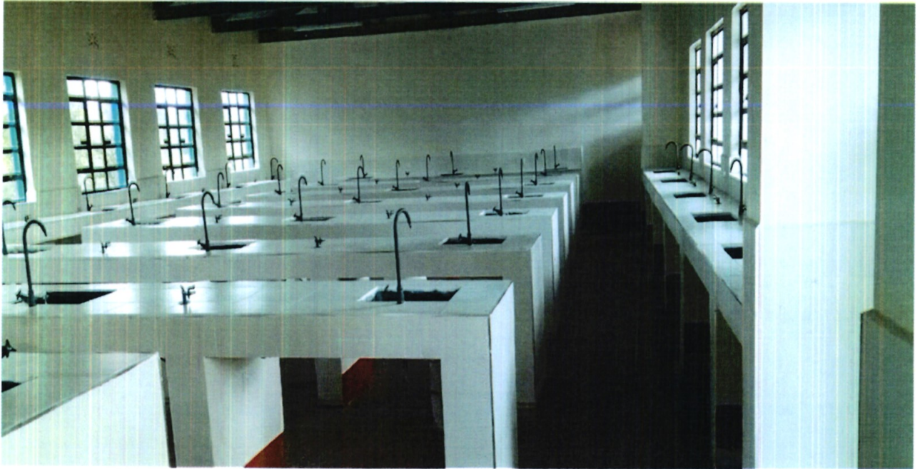
Umoja Secondary School- Ongoing construction of 45 capacity laboratory Laboratory Project
