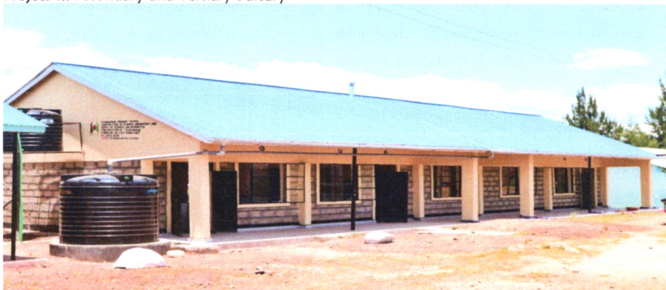
Project 2. Nyamagenga Primary school: Construction of integrated science land, one classroom and supply of laboratory apparatus
