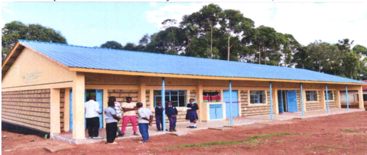
Project 3. Guana Secondary school: Construction of 2 classrooms
