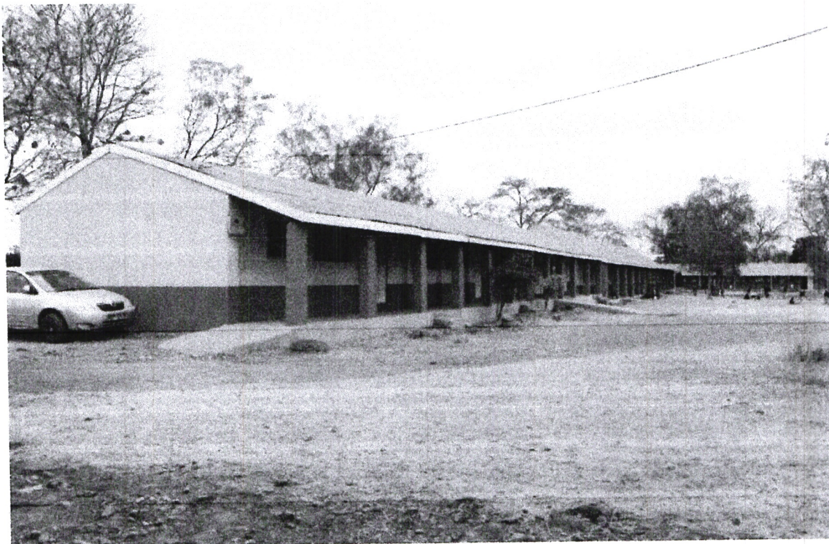
5. Kilimambogo Primary School- Complete renovation of the school
