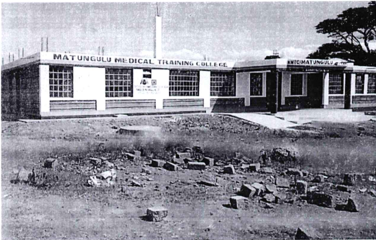
Fig 6 Matungulu KMTTC: construction of administration block
