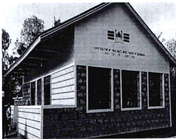
Fig 4 Kingoti chief's office: Construction of chief's office
