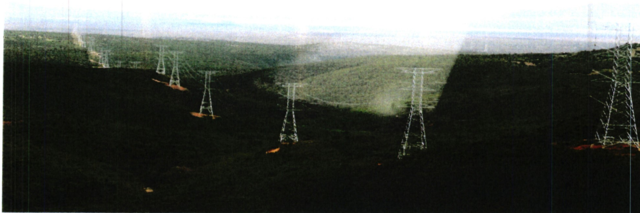
400kV Loiyangalani - Suswa transmission line
