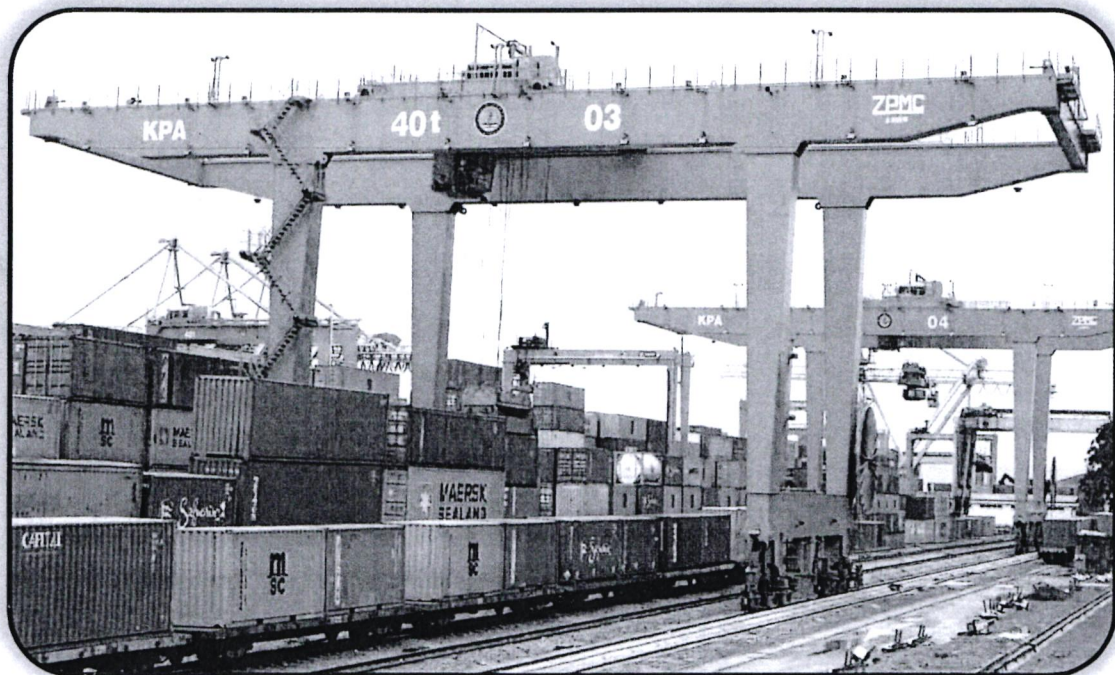
Rail mounted gantries at the terminal
