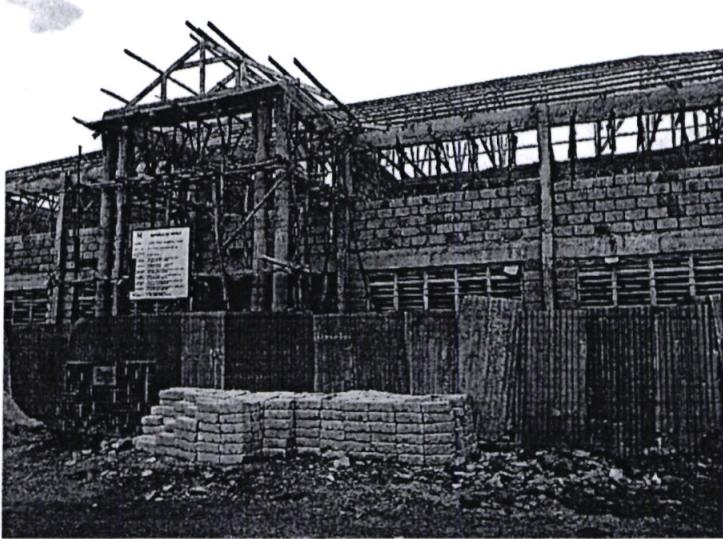
Ongoing Construction of Ainabtich Assistant County Commissioner's office.
