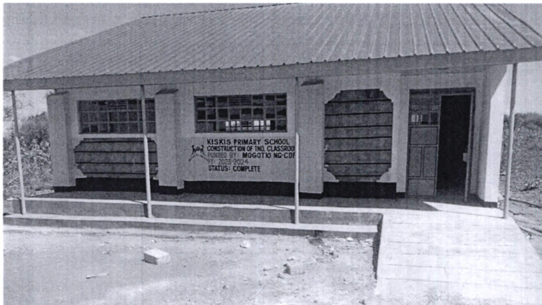
Figure 4-Kiskis Primary School - Construction of One classroom
