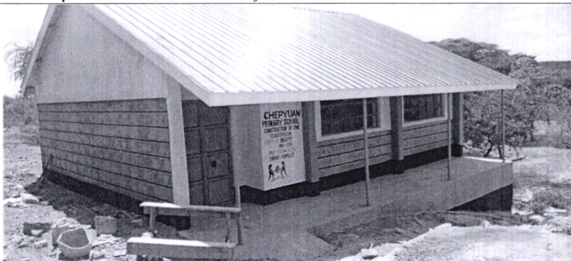
Figure 5 - Chepyuan Primary School - Construction of One Classroom
