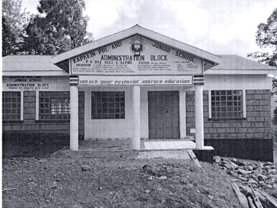
Figure 3-Kapkein Primary school-Construction of Administration Block
