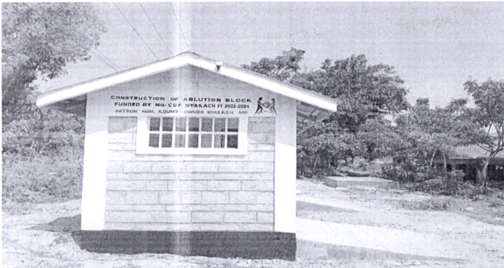
Nyakach Ablution Block
