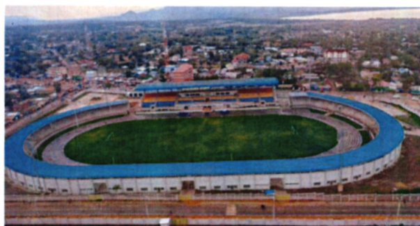
Newly renovated Raila Odinga Stadium that hosted Madaraka Day Celebrations on 1 st June 2025
