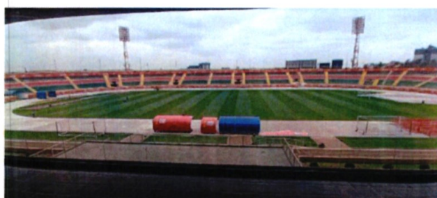
Nyayo National Stadium New look after renovations ready for CHAN 2024 Tournament to be hosted in August 2025
