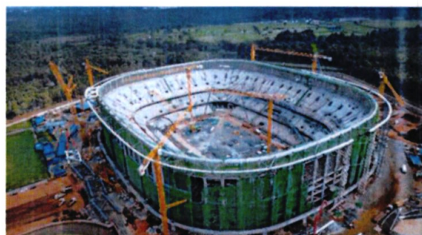
Talanta Sports City Stadium construction on going at 50% stage
