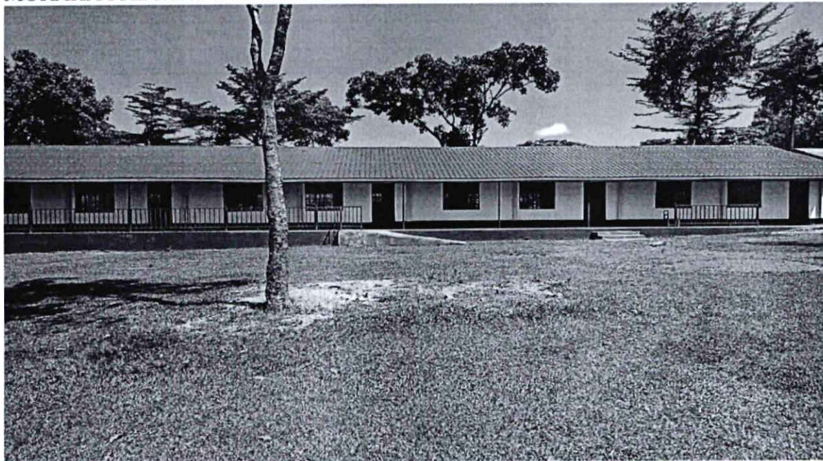
LIRHANDA BORDING PRIMARY SCHOOL FOUR NUMBER CLASSROOMS
