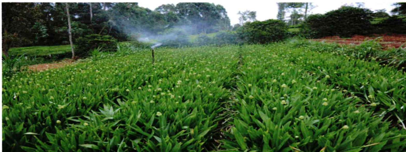
○ Sprinkler Irrigation system in Rwabura Irrigation Project, Kiambu County
