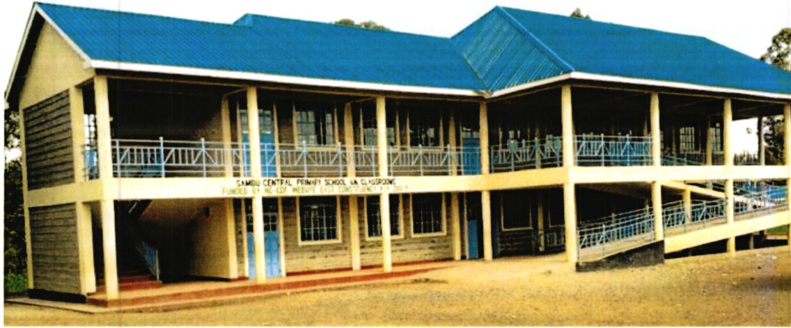
Fig 3: Shows a newly constructed 6 storey classrooms at Sambu Central Primary School in the financial year 2018 – 2019 Webuye East Constituency for enhancing learning environment.
