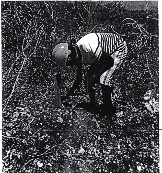
Surveys on establishing the road reserve and chainages
