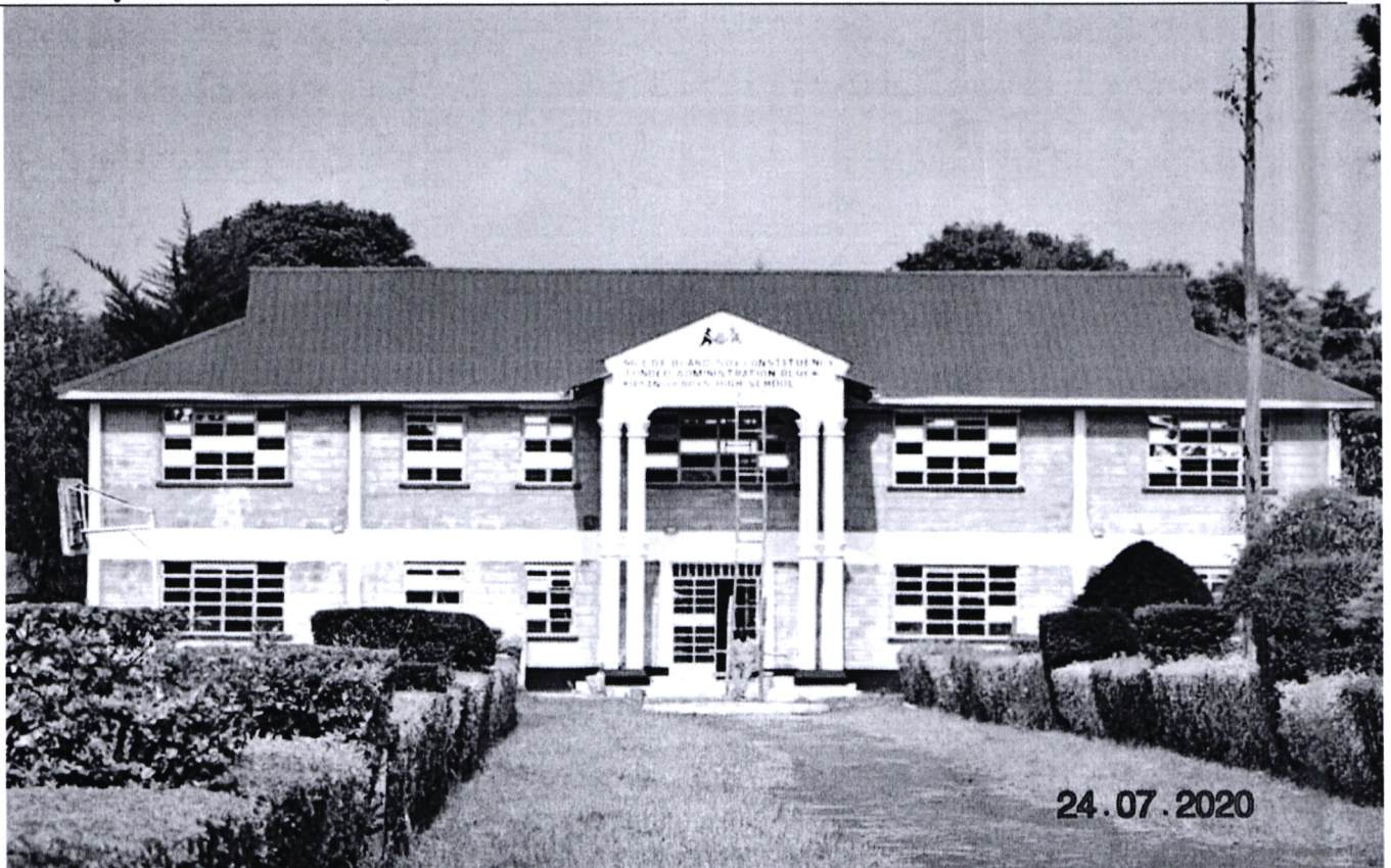
Figure 6. Kipsangui Boys High School completion of administration block at Kshs. 8,000,000.
