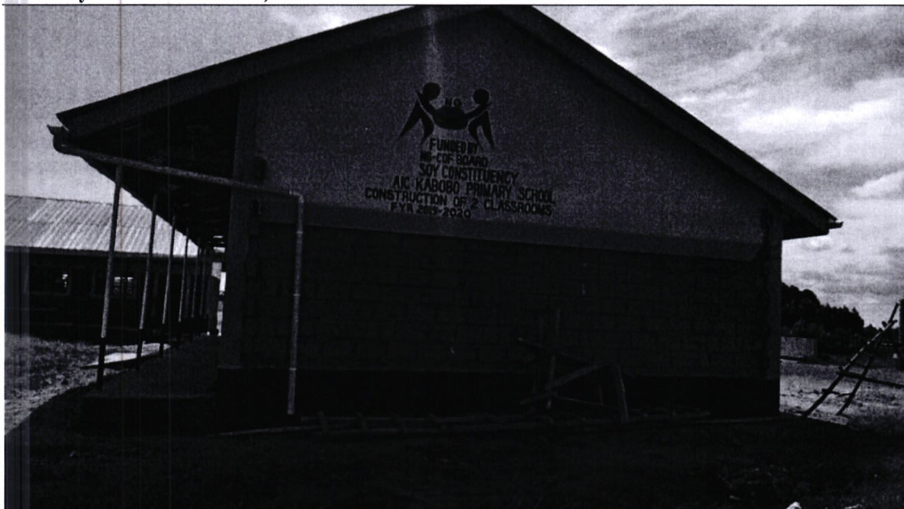
Figure 8. AIC Kabobo primary school construction of 2 classrooms at Kshs. 1,700,000
