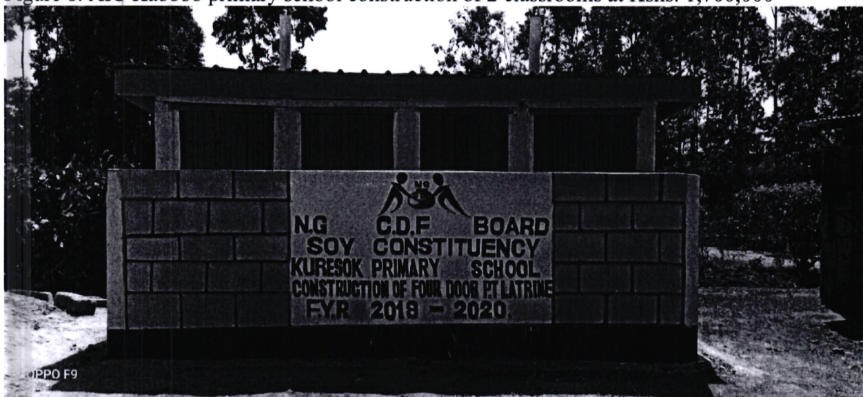
Figure 6. Kuresok primary school construction of 4 door pit latrine at Kshs 250,000
