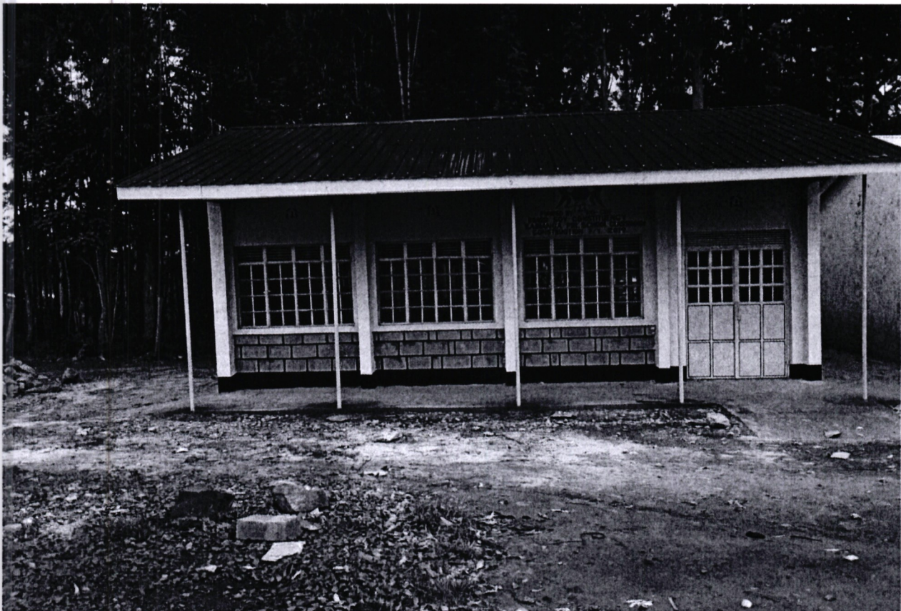
Figure 1. Kabianga sisal primary school Construction of 1 classroom at Kshs 850,000
