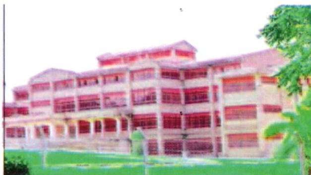
Ongoing construction of Library and Administration Block
