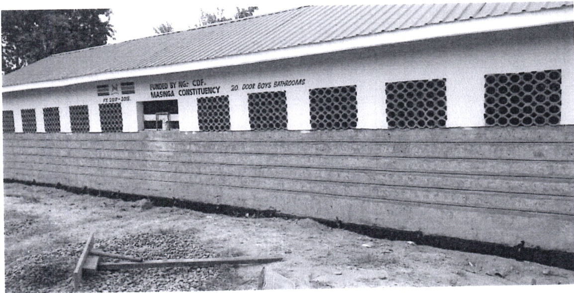
Back View Bathrooms
