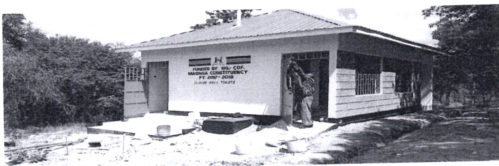
Girls Toilets – Kivaa Secondary School
