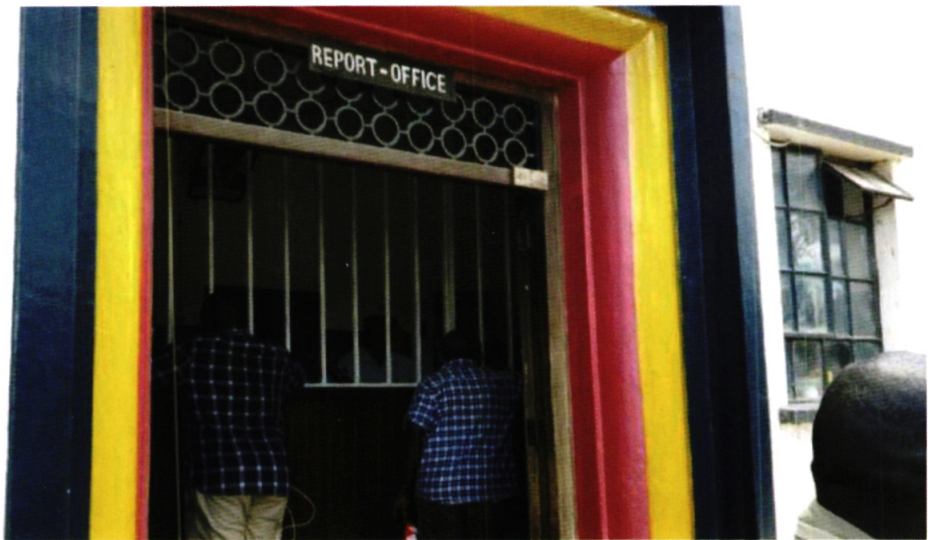
Photo: A Grilled Report office in Sultan Hamud Police Station for security purposes
