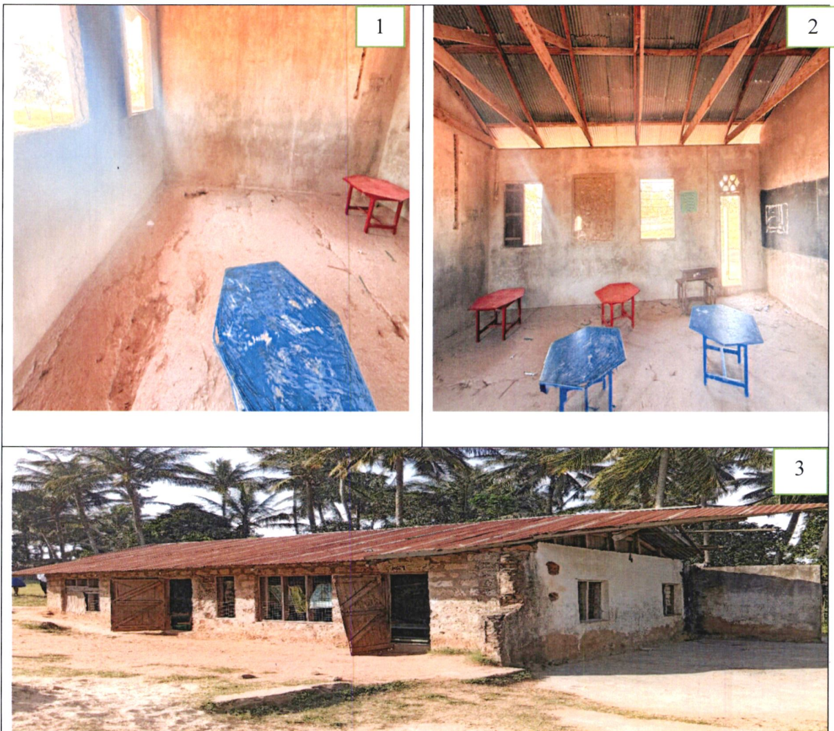
Picture 1 and Picture 2 : Showing dilapidated floors and classroom without window panes and doors at Bamba Pre-primary School, Picture 3 Showing dilapidated walls and roof at Chanagande Pre-Primary School
