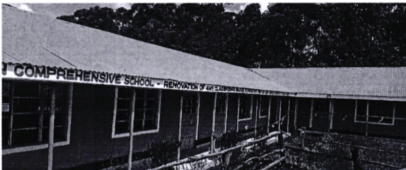
Emdin primary school Renovation of 4 No classrooms
