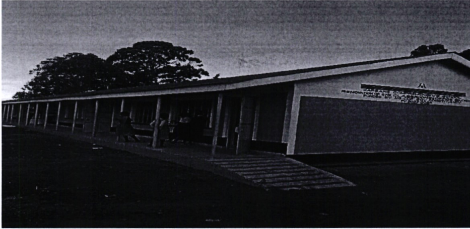
Renovated 5No classrooms at Kapsang primary
