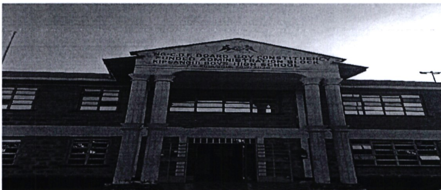
Complete single storey administration block at Kipsangui boys High school
