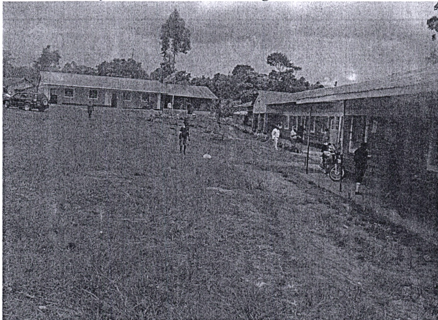
Pic. 1: Muyere Secondary School newly constructed 6No. classrooms and an administration block fully funded by Hamisi NG-CDF
