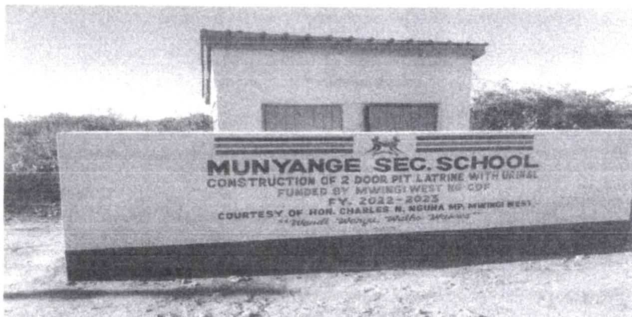
FIG 1.3: Two door pit latrine constructed at Munyange Secondary School, completed FY 2022/2023 to improve students' sanitation conditions.
