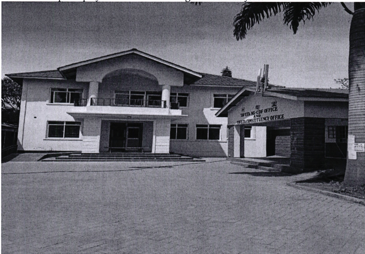
a. Extension of Ng-CDF Office- Ongoing
