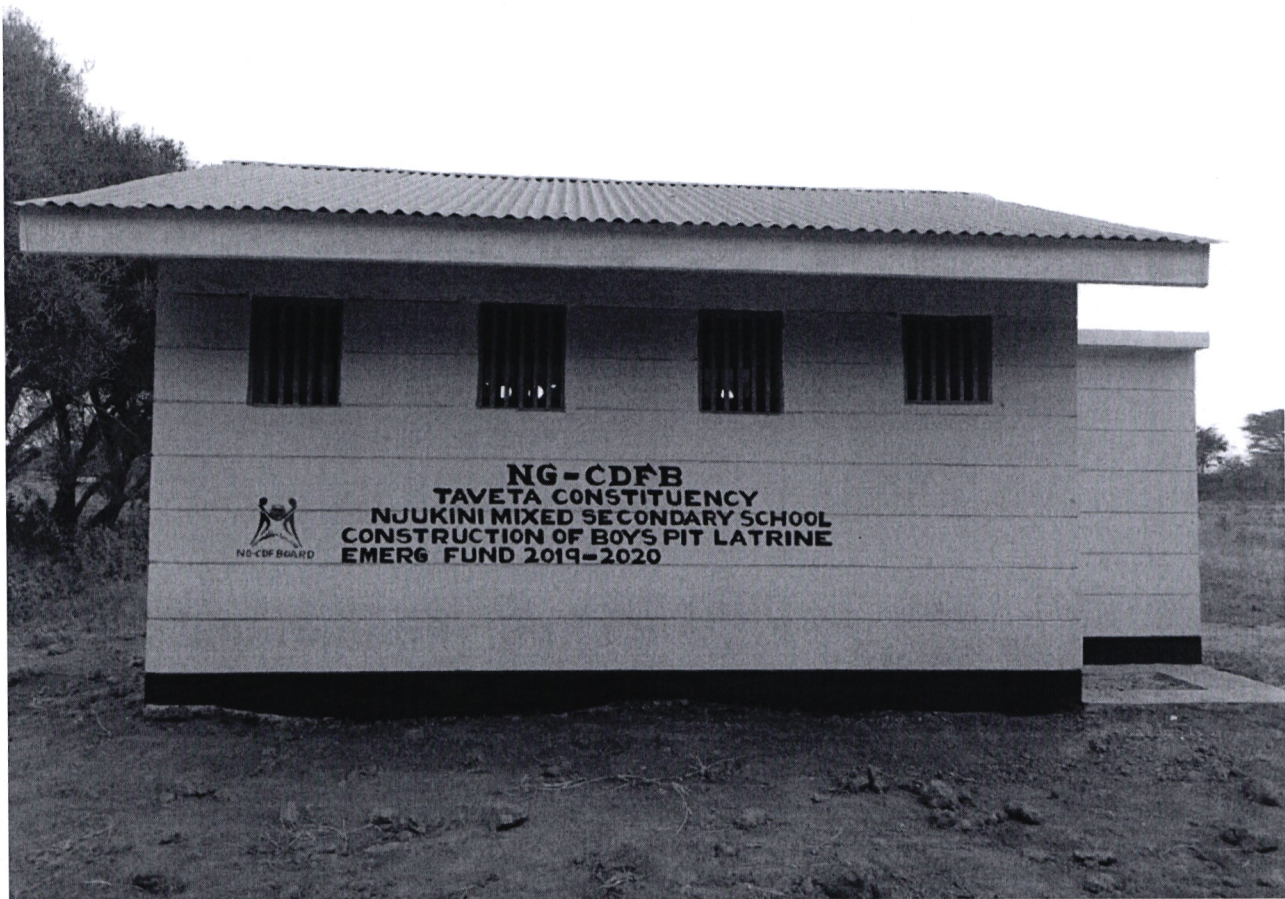
h) Construction of pit latrine at Njukini secondary school- complete
