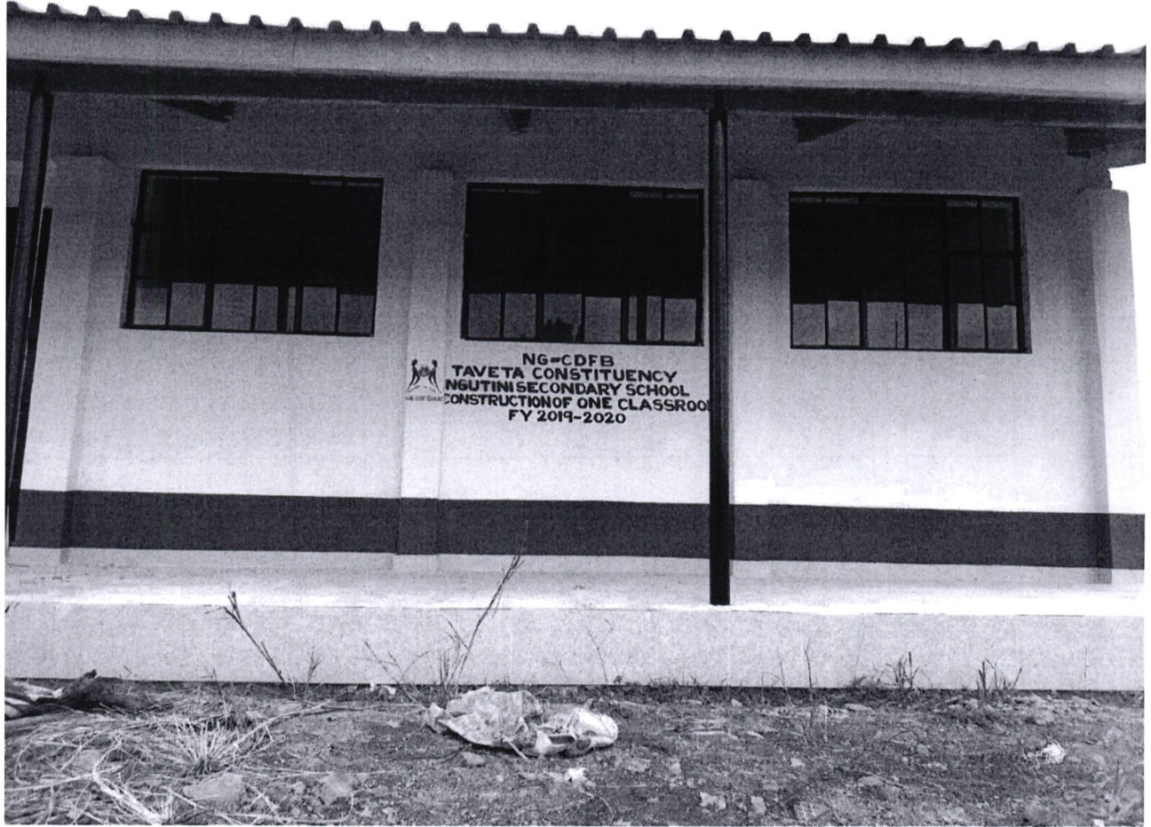
c. Construction of one complete classroom at Ngutini secondary school
