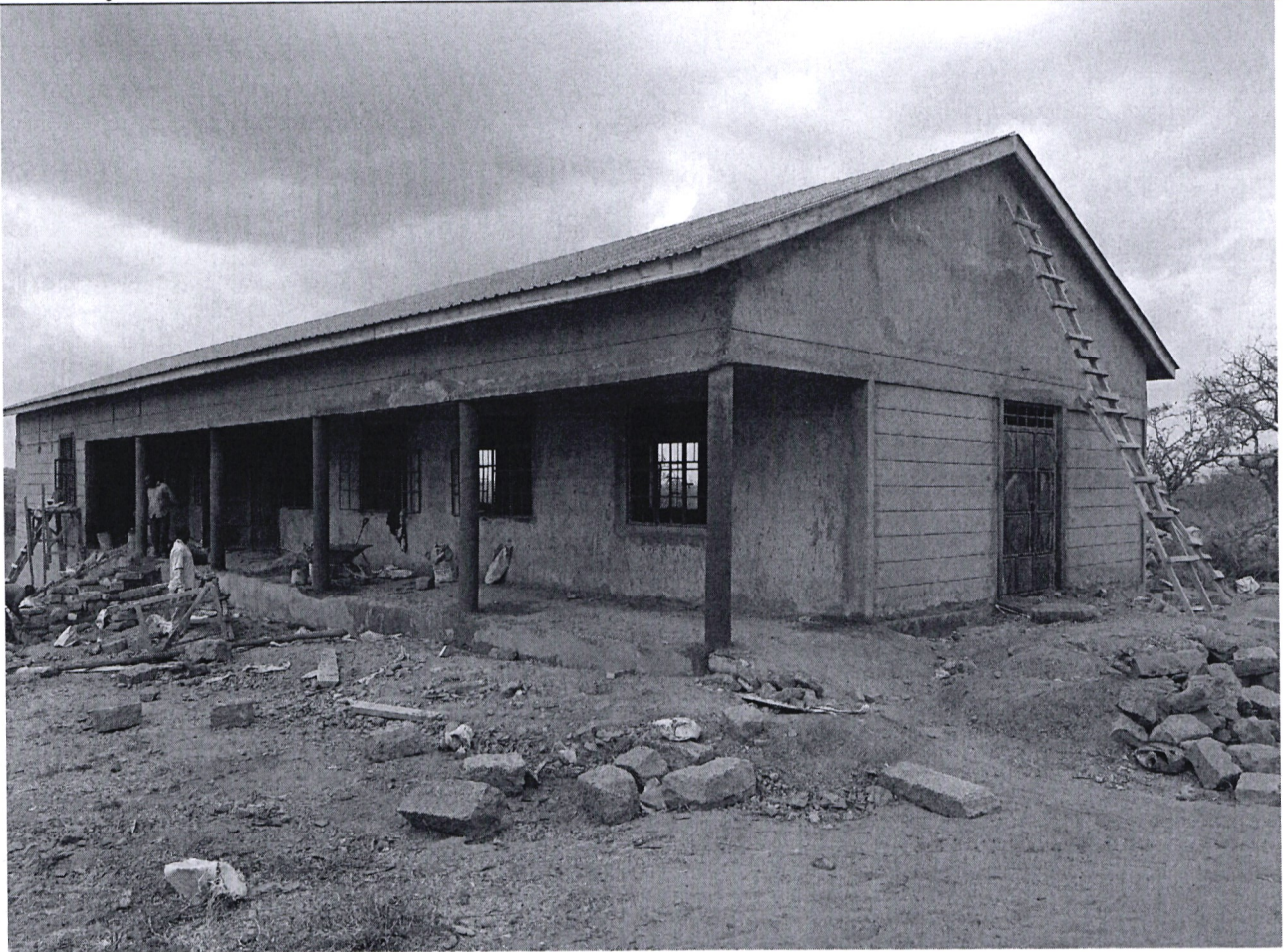
b. Construction of Nakruto Chief's office- Ongoing
