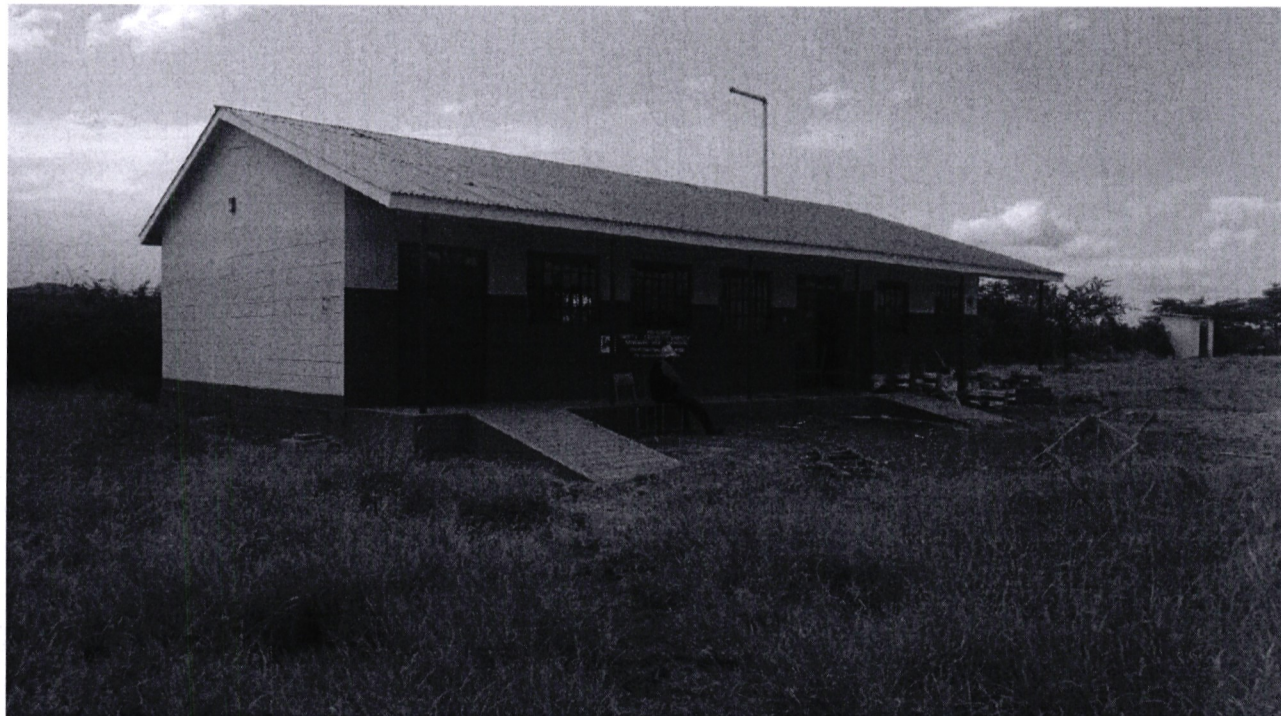
g) Construction of laboratory at Sowene secondary school- complete
