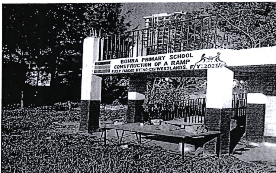
Fig 4: Construction of a Ramp at Bohra Primary School
