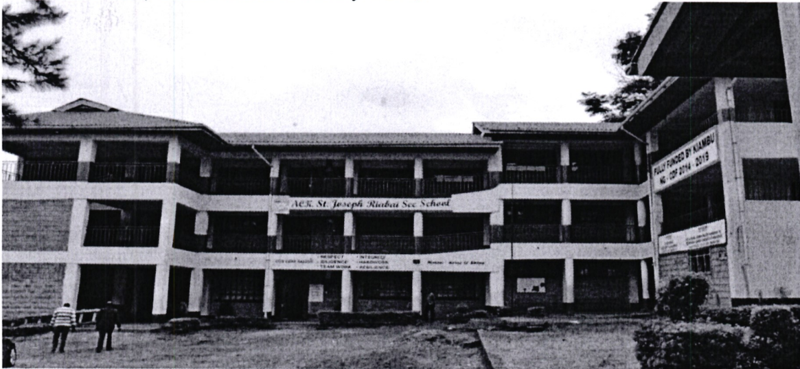
St Joseph Riabai secondary school- complete project (Administration, classrooms and library block)
