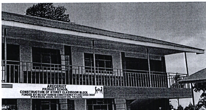
Project 3: Aregeriot primary School construction of 4NO storey classrooms.
