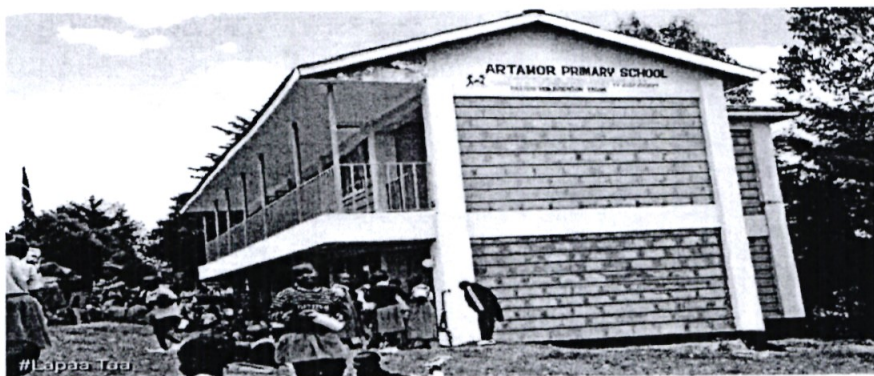
Project 2: Artamor Primary construction of 4NO storey classrooms.
