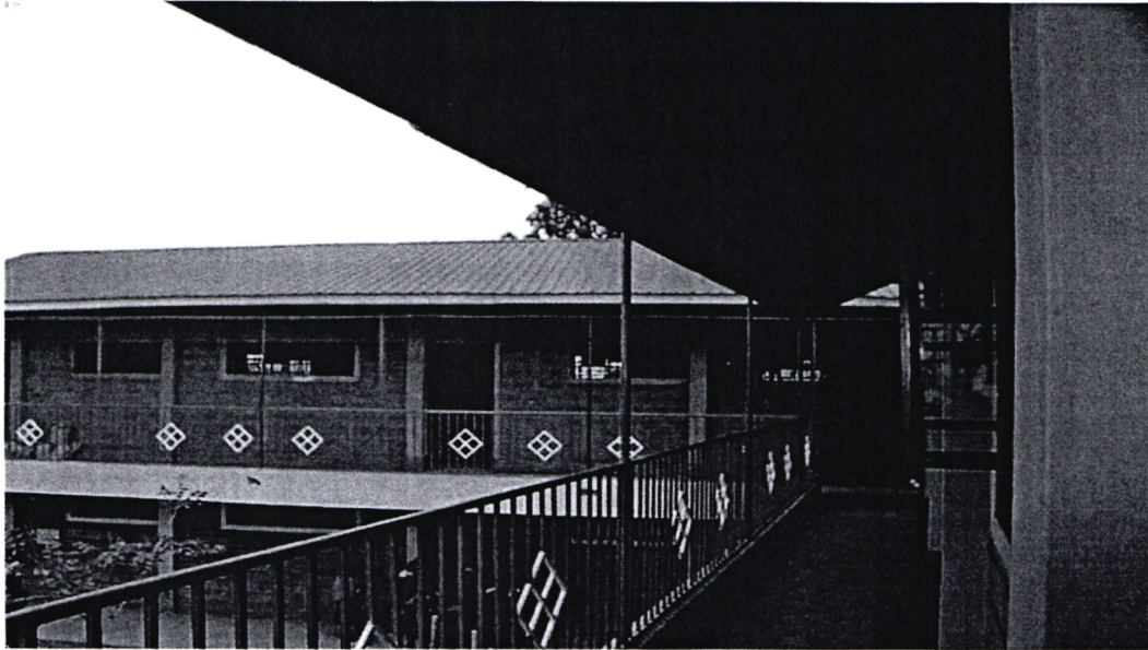
Njathaini Primary School: Construction of an additional 2No. Classrooms
