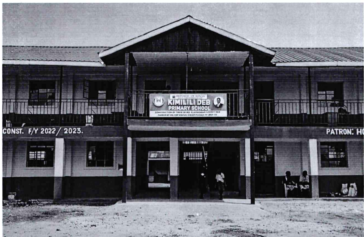
Kimilili D.E.B Primary school Construction of 8No classrooms. FY 2022/2023
