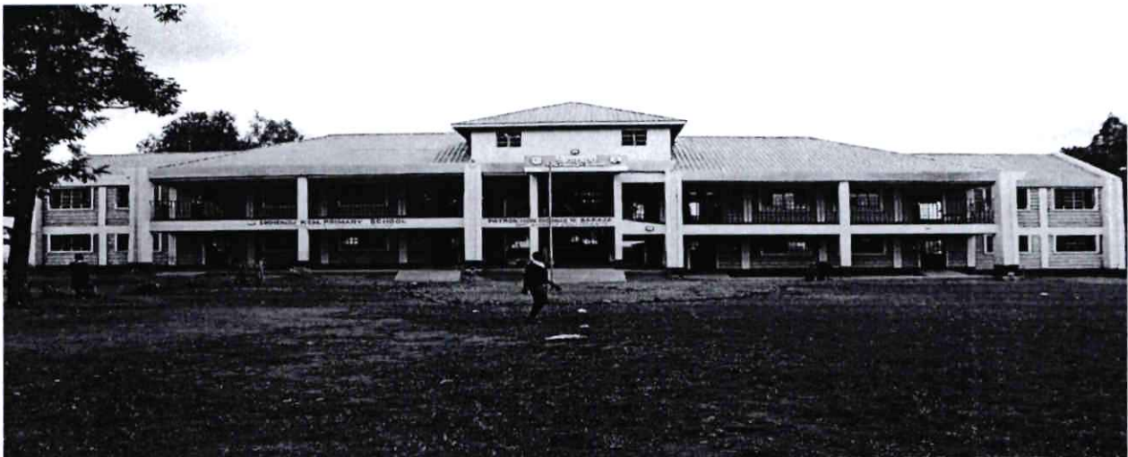
Sikhendu FYM Primary School. Construction of 8No classroom. FY 2022/2023
