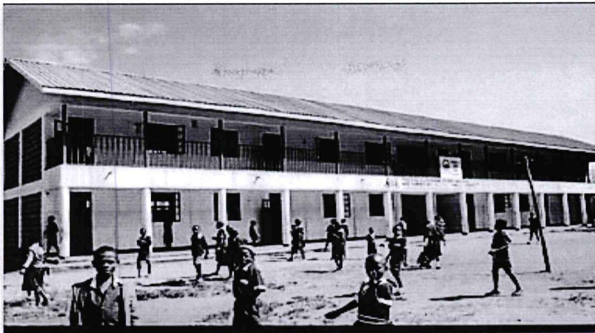
Chesamisi FYM Primary School Construction of 8No classroom FY 2022/2023
