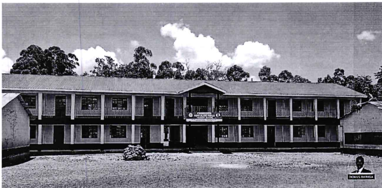
Kimilili R.C Girls –Construction of 8No classroom FY 2022-2023
