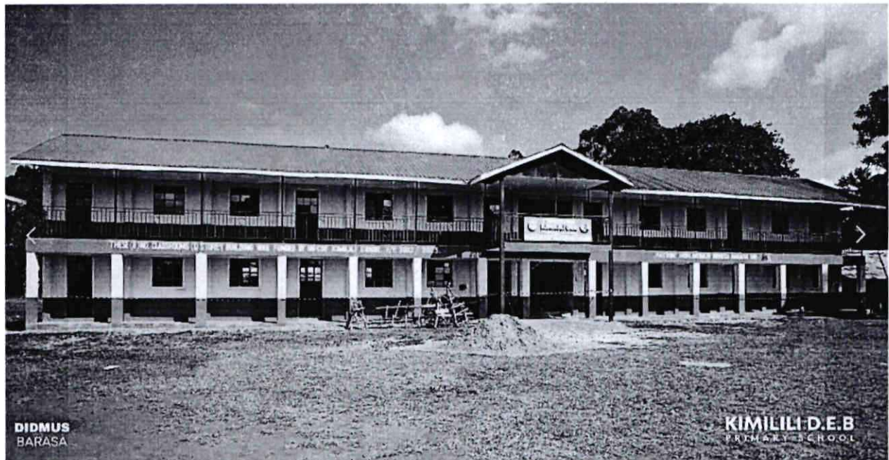
Kimilili D.E.B Primary school Construction of 8 No classrooms - FY 2022-2023
