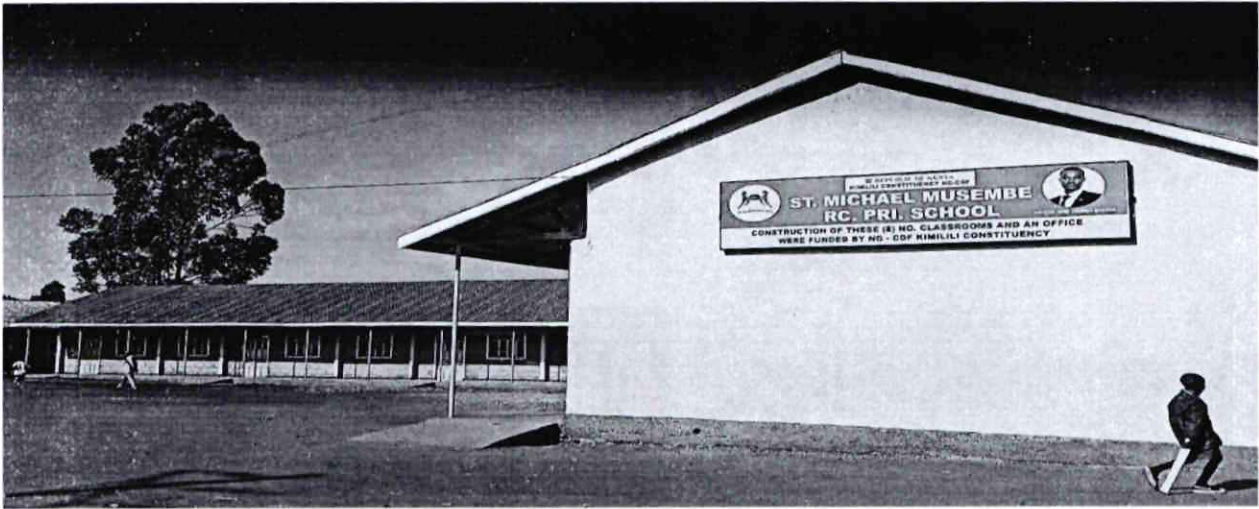
St. Michaels Musembe R.C Primary School Construction of 8 No classrooms-FY 2022-2023
