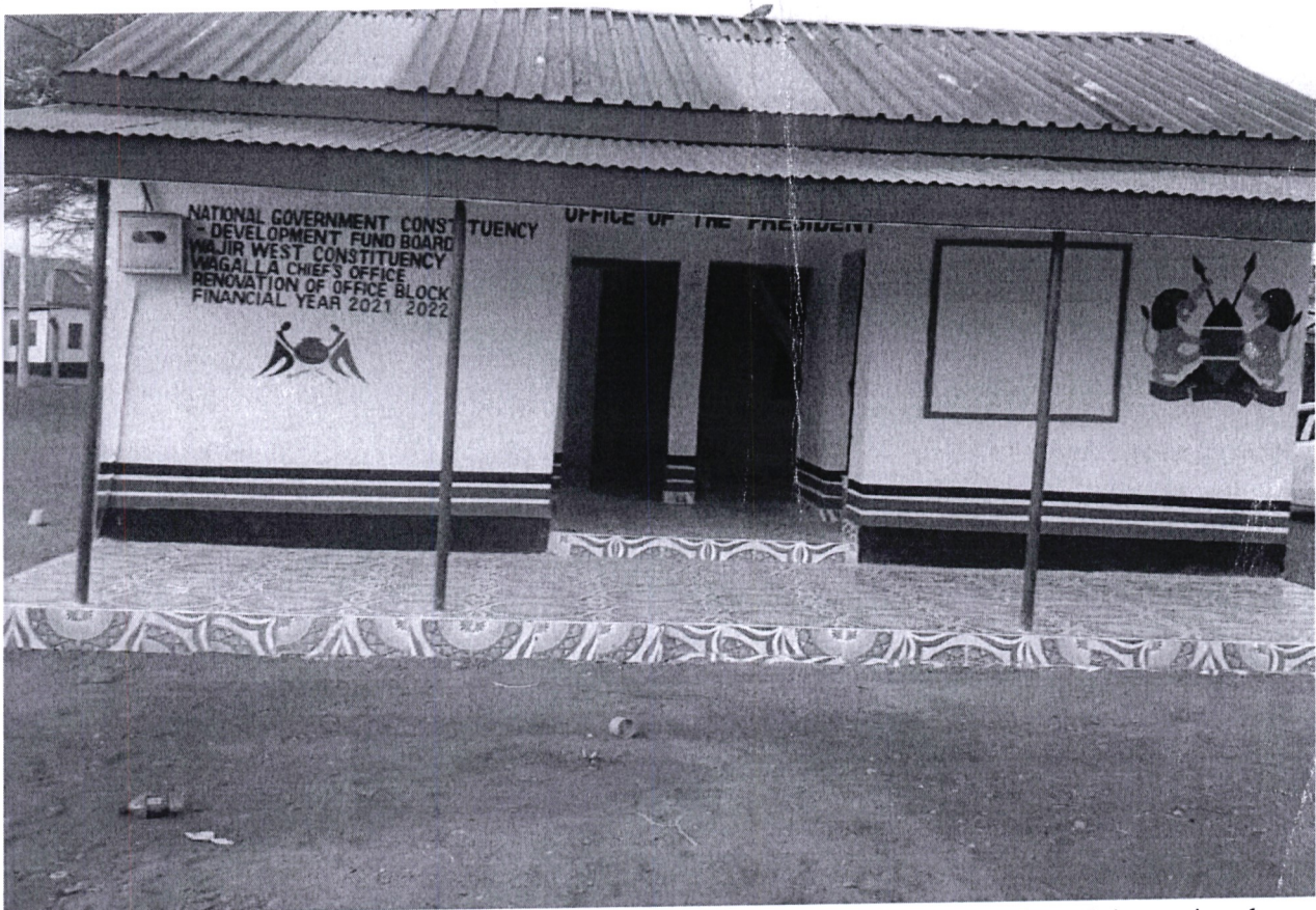
This is Wagalla Chief's office in Wagalla town. Wajir West constituency NGCDF has funded the project to bring services closer to the people and improve security in the location.
