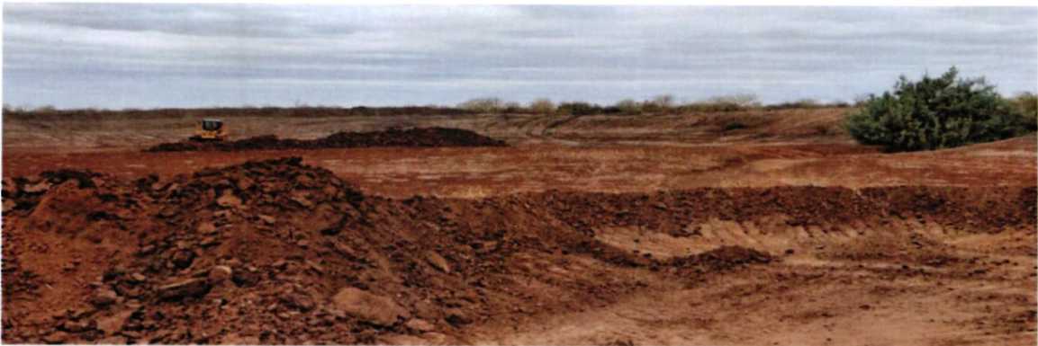
Photo 2: Clearing and deepening of the water pan bed.
