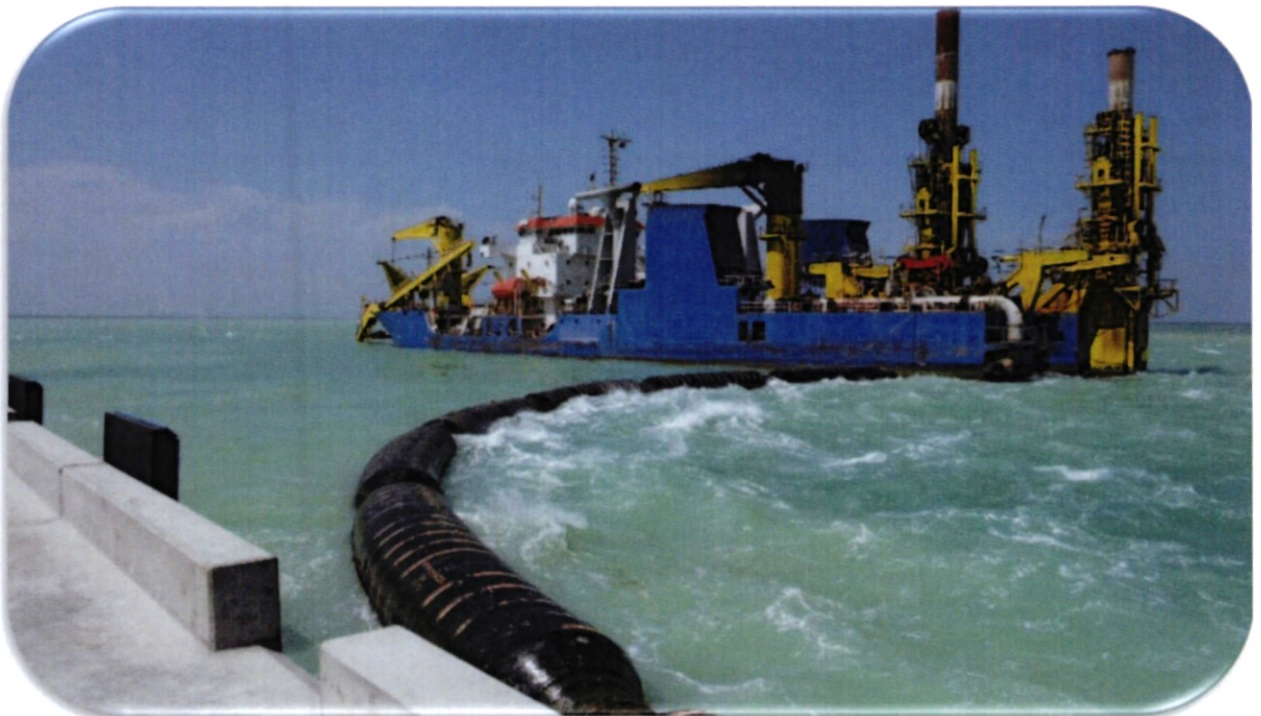
Figure 2: Dredging channels at the Port of Lamu
