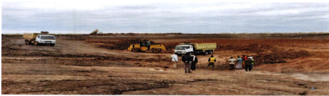
Photo 1. Community members observe the excavation works.
