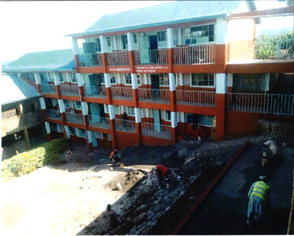
On going paint works and landscaping
