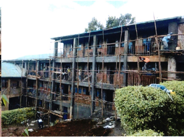
Plastering columns & beams externally on going
