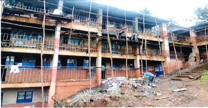
External plastering on columns and beams.
