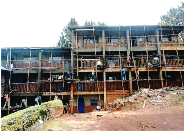
Plastering columns & beams externally on going
