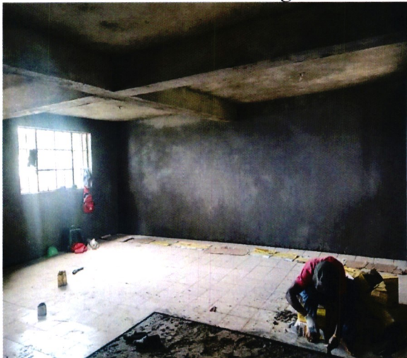
Classroom Floor tiling and Staffroom on going.
