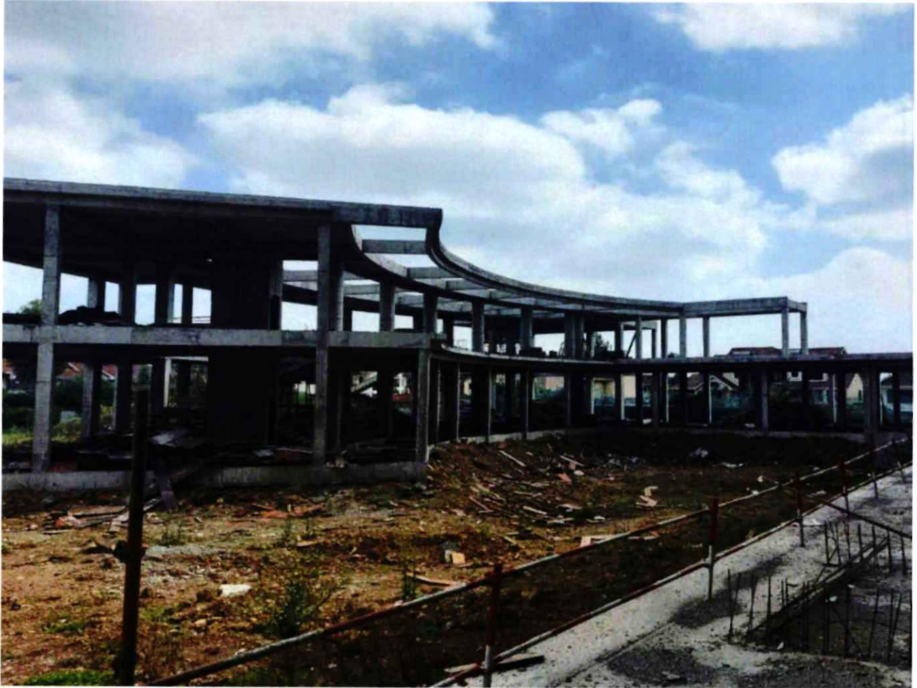
Figure 6: Ongoing CPST Construction Project
