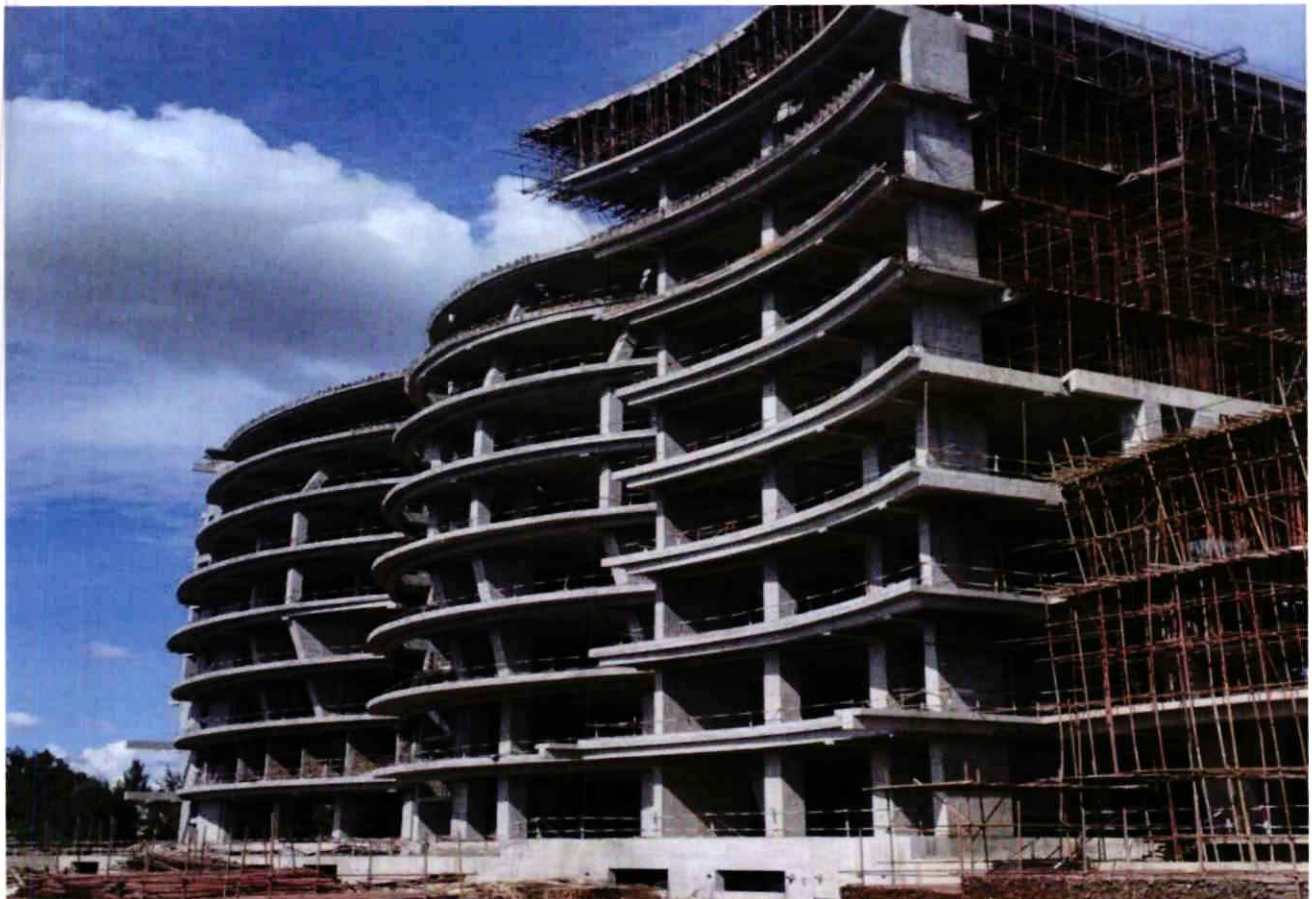
Figure 5: Ongoing CPST Construction Project
