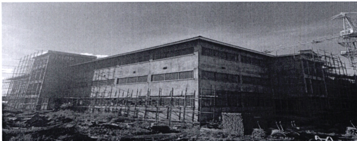
Figure 4. Ongoing Construction of modern market
