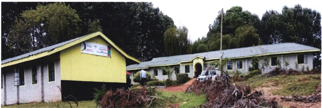
❖ NGURWEINI PRIMARY SCHOOL CLASSROOMS RENOVATED BY KIGUMO NG-CDF
