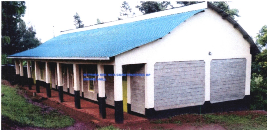
❖ GITHIMA PRIMARY SCHOOL MULTI PURPOSE HALL CONSTRUCTED BY KIGUMO NG-CDF
