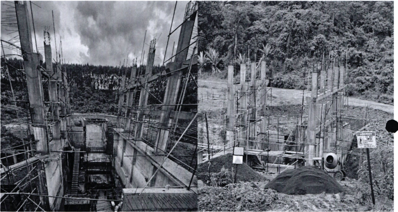
Powerhouse under construction
