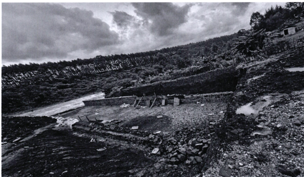
Spillway under construction
