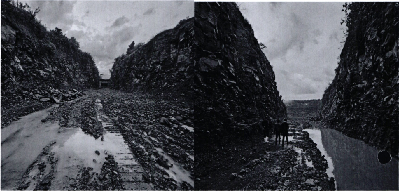
Part of the Canal Blasted under construction
