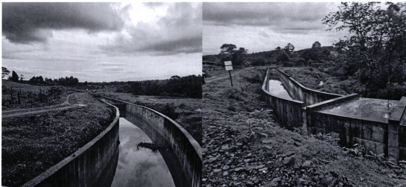
Completed part of the Canal
