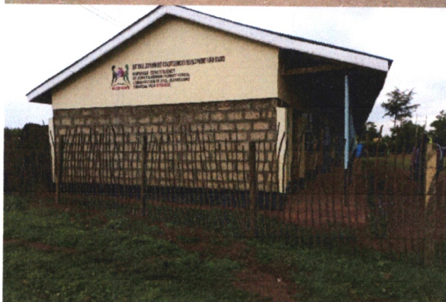
Figure 4: Completed 2no. classrooms at Kimalael primary
