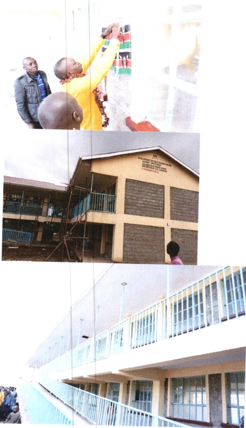
Figure 2: commissioning of the completed 12no. classrooms at Kipkaren Road Primary School
