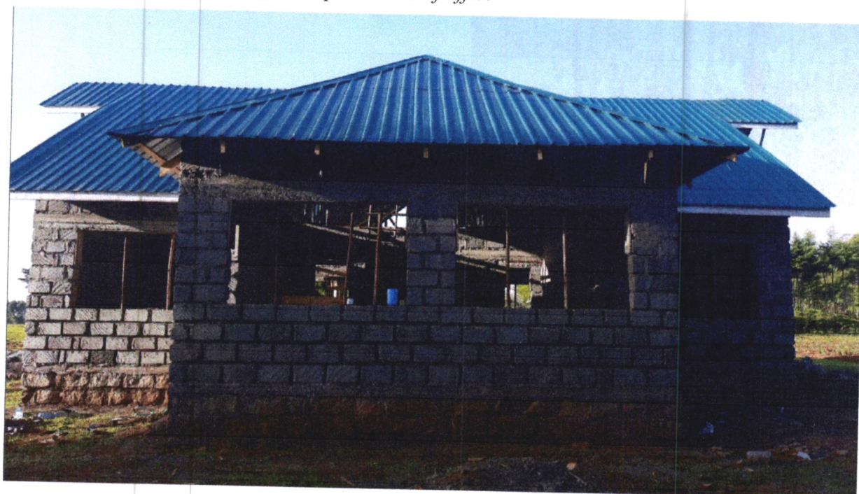
Figure 1: Ongoing construction of assistant chief's office at Megun assistance chief office
