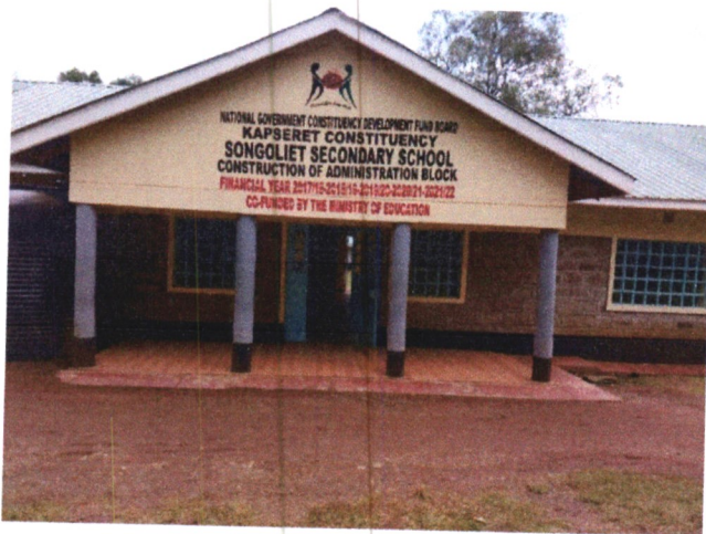
Figure1: Construction of Administration Block at Songoliet Secondary School
