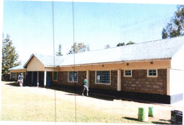
Figure5: Completed 2no.C lassrooms at St. Johns Kabongo pri. sch
