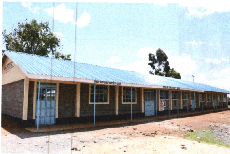
Figure 3: Complete 3no. Classroom Mwiruti secondary school
