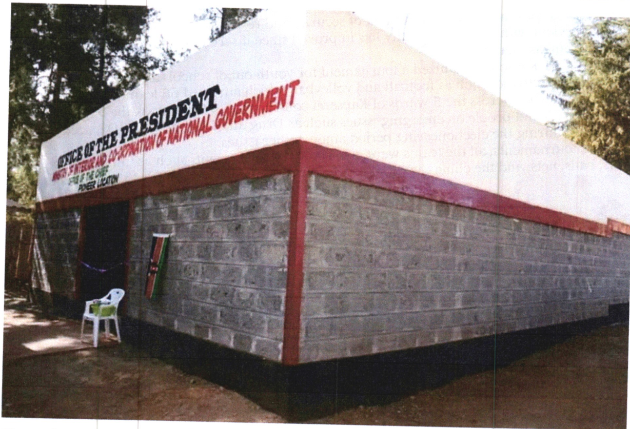
Figure 1: complete chief's office at pioneer chief office
