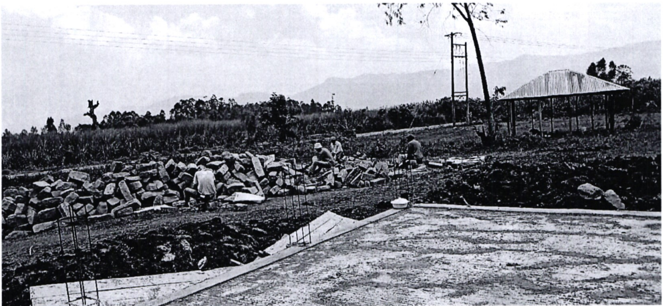
On going construction of Orege Secondary School
